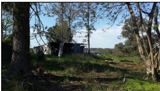
Dilapidated Outbuilding, to be demolished
