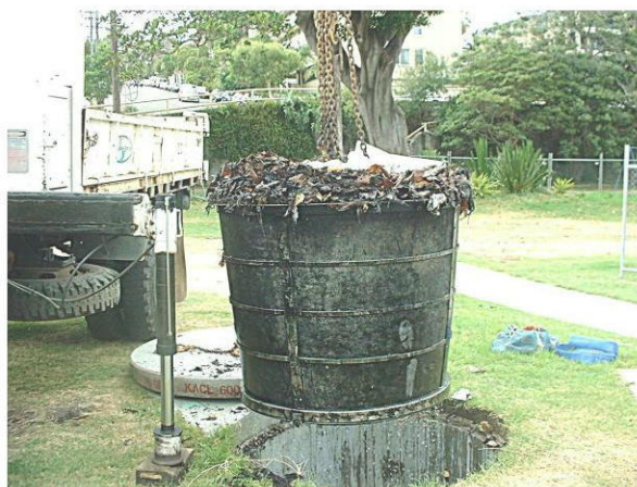
PLATE 6.1 EMPTYING THE BASKET CONTAINING THE SOLIDS IN A WET SUMP GPT
