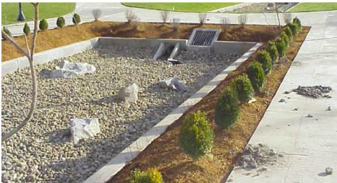
PLATE 6.4 SAND FILTER
