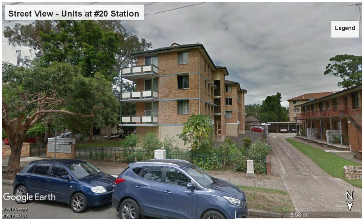
Figure 15 Image showing existing four storey residential flats at #20 Station Lane (to the immediate north of the subject site) (image courtesy of Google Earth Pro)
