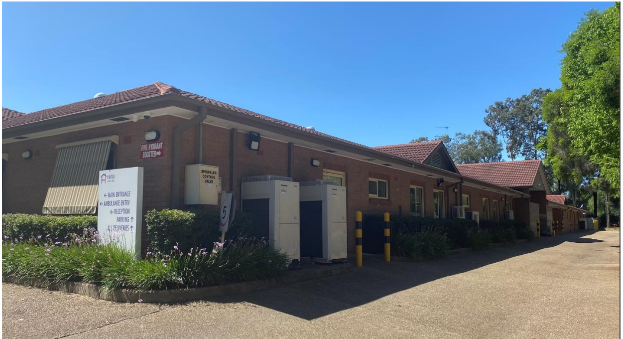
Figure 4 Southern side of the dwelling on the subject site.
