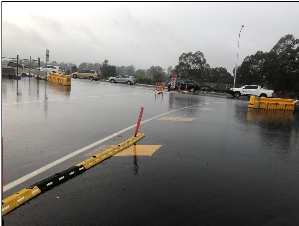
Figure 4c: Stop intersection of The Northern Road with Garswood Road
