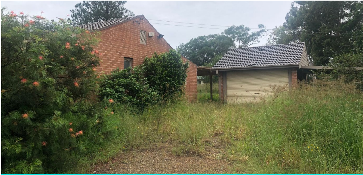
Figure 6 – Existing vehicle entry (Corona Projects, 2020)
