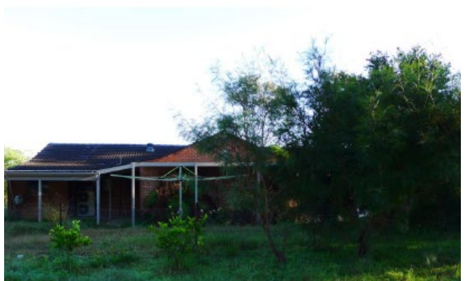
Photo 6 – The existing house
