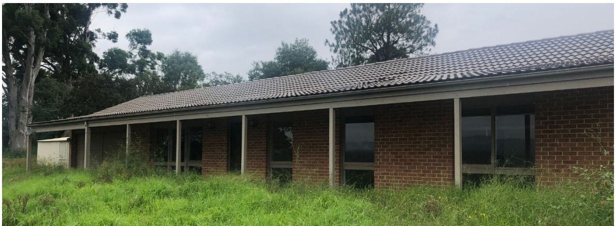
Figure 5 – Existing main building (Corona Projects, 2020)
