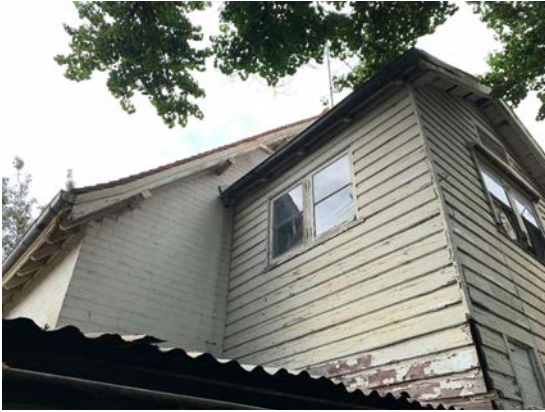
Figure 9: View of the southwestern elevation.
