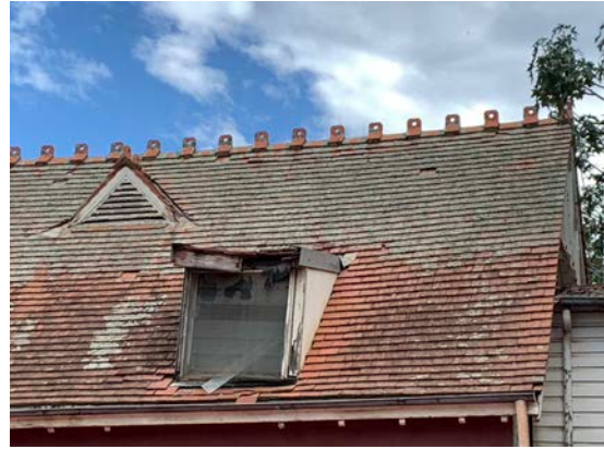
Figure 10: View of the eastern roof plane and dormers.
