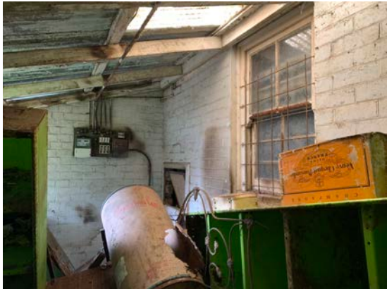
Figure 15: View of the semi-enclosed verandah on the western elevation.
