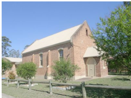
Figure 43: St Phillip's Anglican. [Source: NSW State Heritage Inventory, 2020]
