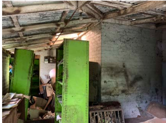
Figure 16: View of the semi-enclosed verandah on the western elevation.
