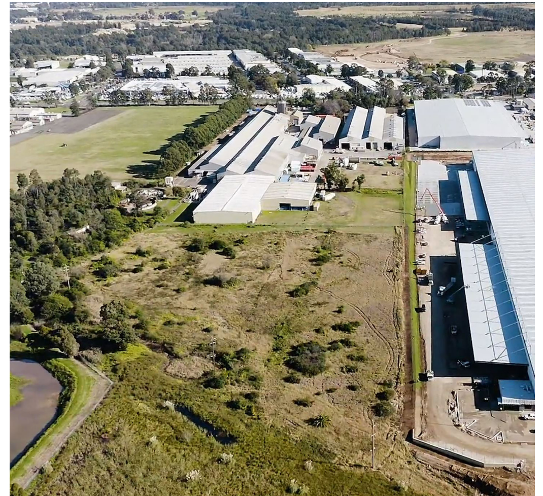
02 - Aerial View Looking West
