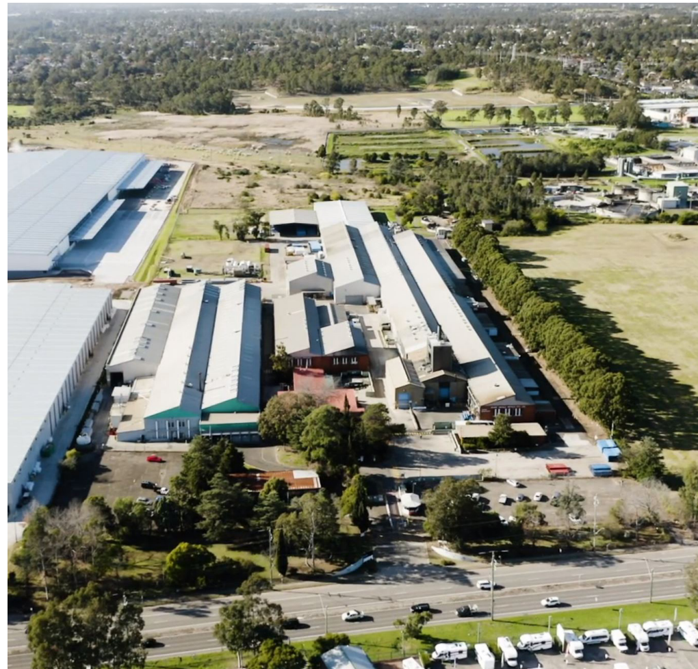
01 - Aerial View Looking East
