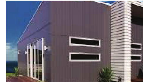
F1: 7.5MM MIN. THK F.C. SHEET, RENDERED DULUX 'BEIGE ROYAL HALF' P15B1H
