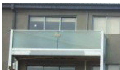
OG: BALCONY BALUSTRADES. OBSCURE GLAZING (OR TRANSLUCENT)
