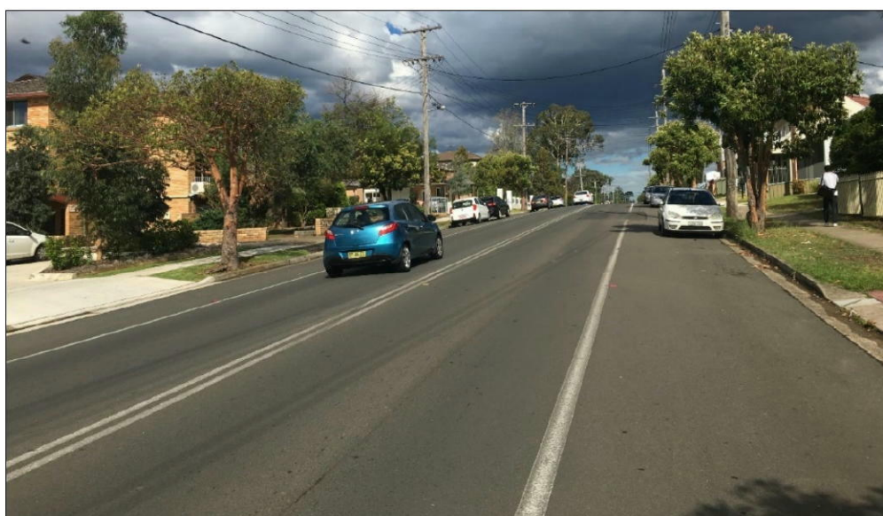
Figure 6: Derby Street facing East
