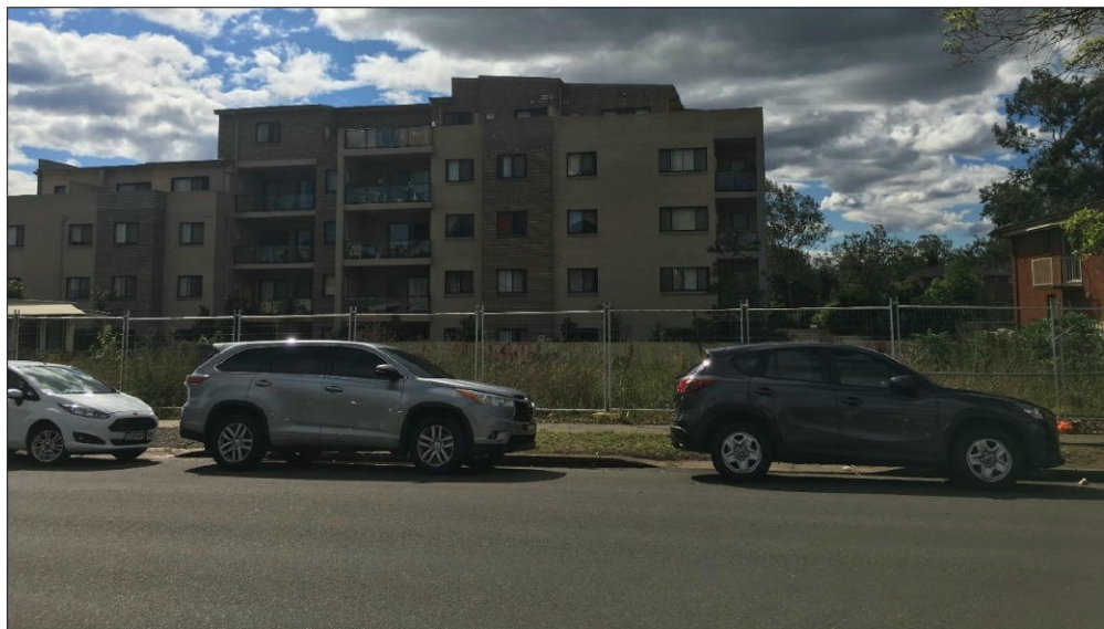
Figure 3: Photograph of 29-31 Castlereagh Street in Penrith
