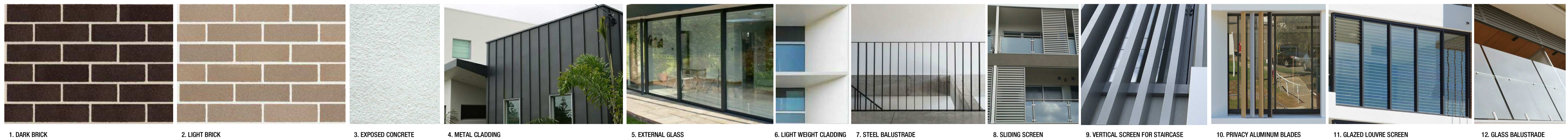
1. DARK BRICK 2. LIGHT BRICK 3. EXPOSED CONCRETE 4. METAL CLADDING 5. EXTERNAL GLASS 6. LIGHT WEIGHT CLADDING 7. STEEL BALUSTRADE 8. SLIDING SCREEN 9. VERTICAL SCREEN FOR STAIRCASE 10. PRIVACY ALUMINUM BLADES 11. GLAZED LOUVRE SCREEN 12. GLASS BALUSTRADE
