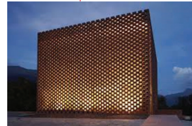
Wall wash light effect to amenities building side facade
