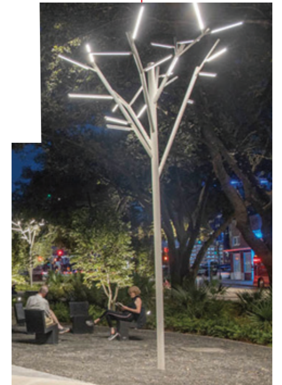
Light poles within grove of trees
