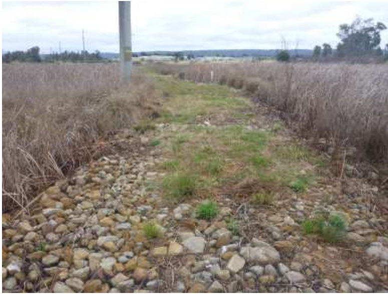
Plate 15 Electrical easement and raised track within the swampy area in the south-eastern portion of the study area, featuring pebbles overgrown with grass, facing south-west
