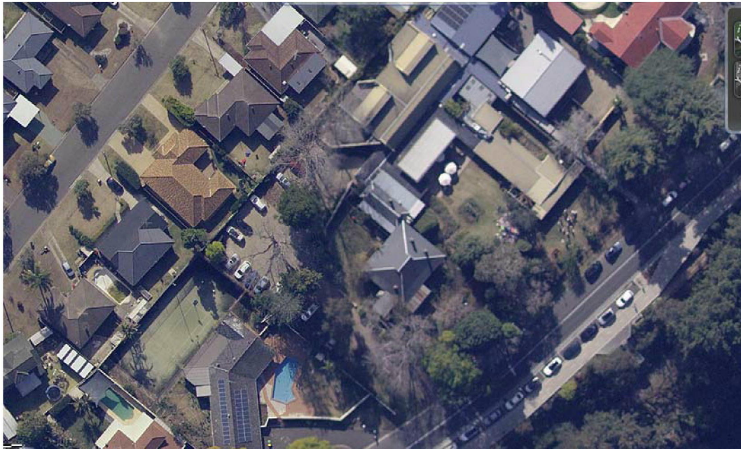
Aerial of 84-88 River Road , illustrating edge of boundary defined by solid structure. Extract: NSW Land Titles Six maps 23.9.2019
