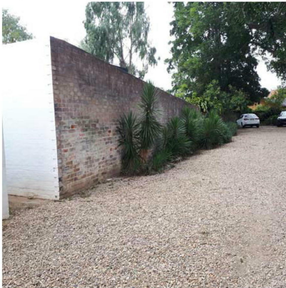
Carpark South east view – Succulents on western face of common wall with Lewers Courtyard.
