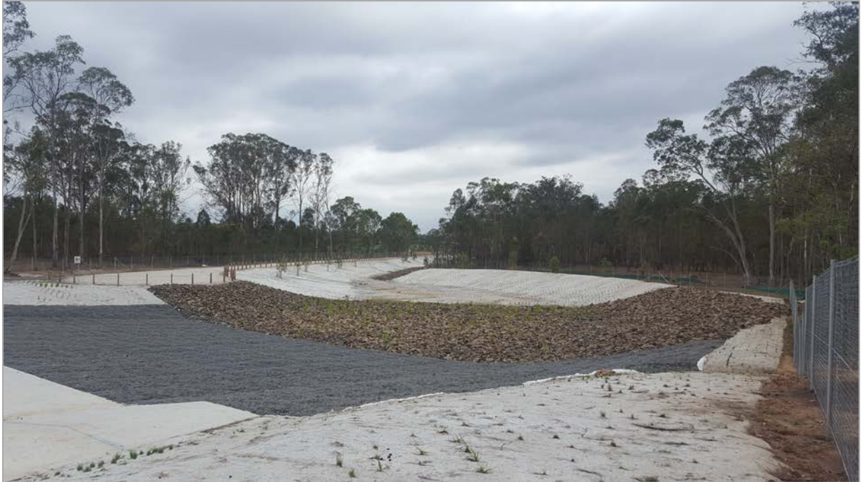
Photograph 3: Stormwater basin and perimeter maintenance road along southern interface
