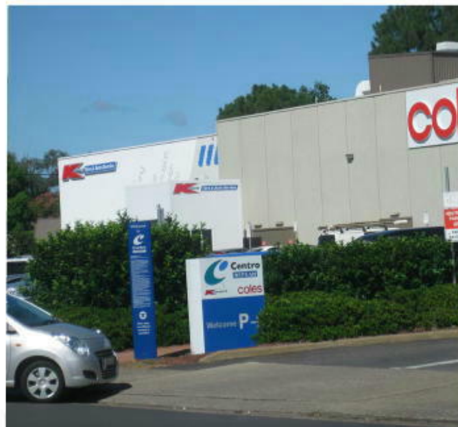
EXISTING CONDITIONS - SIGN 8 (NTS)
