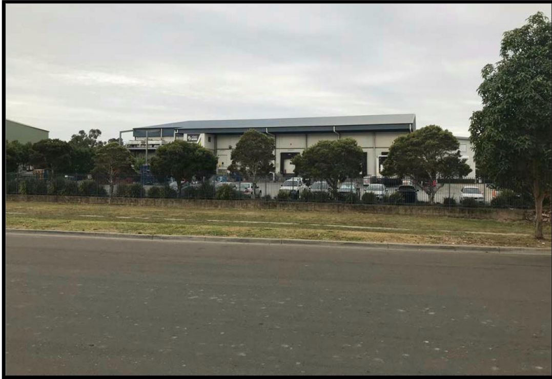
Photograph 4 – View of site looking east.
