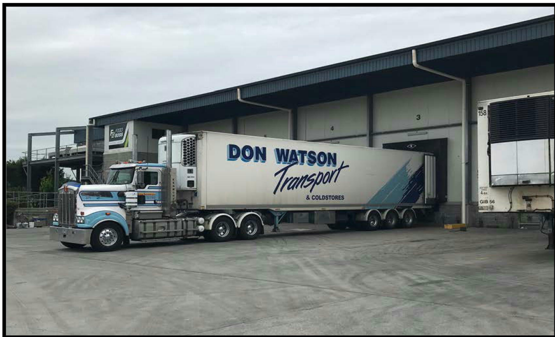
Photograph 3 – View of loading area.
