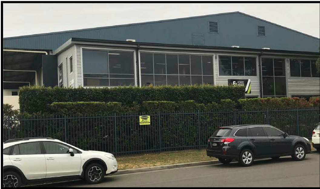
Photograph 2 - View of existing premises administration fronting Lambridge Place.
