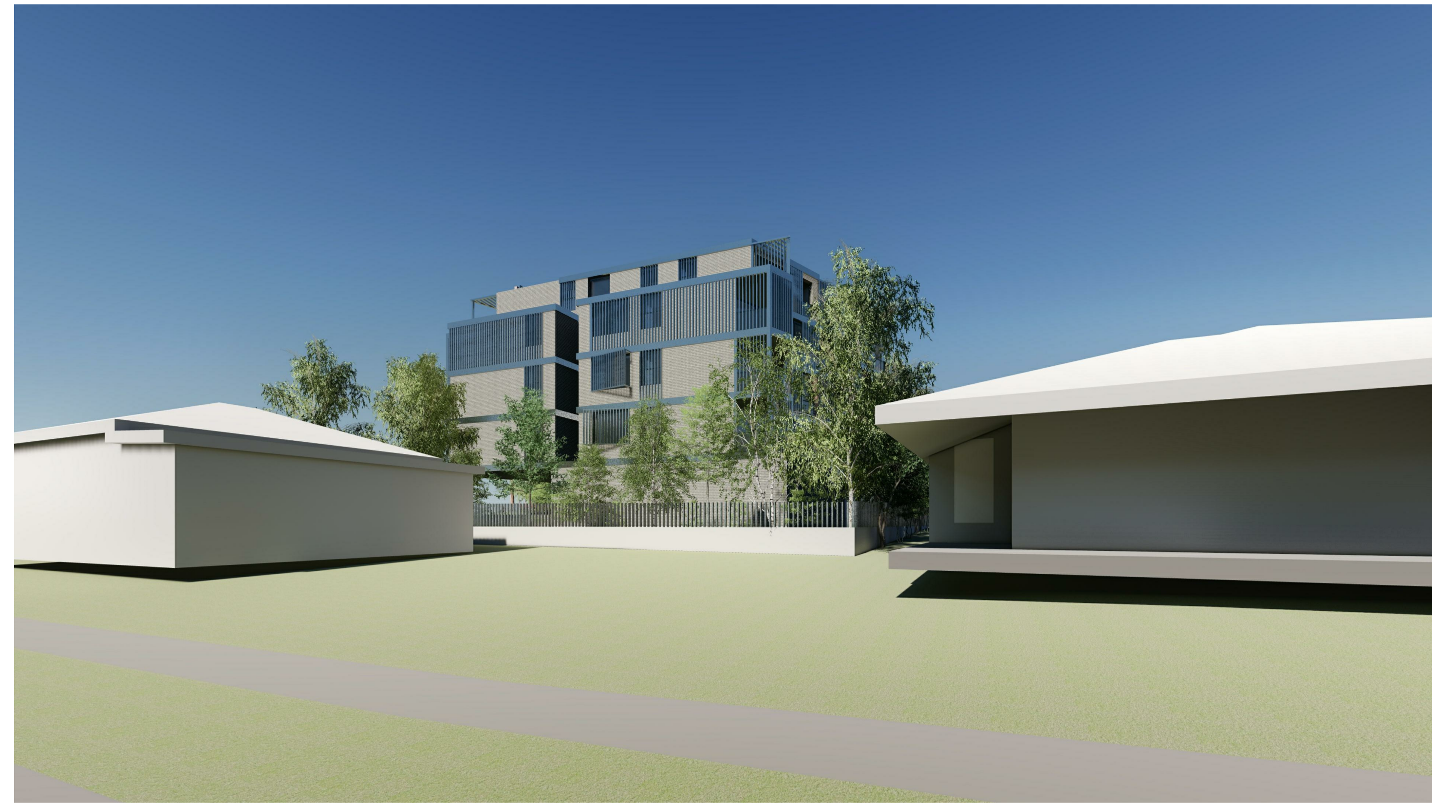
VIEW FROM LETHBRIDGE ST
