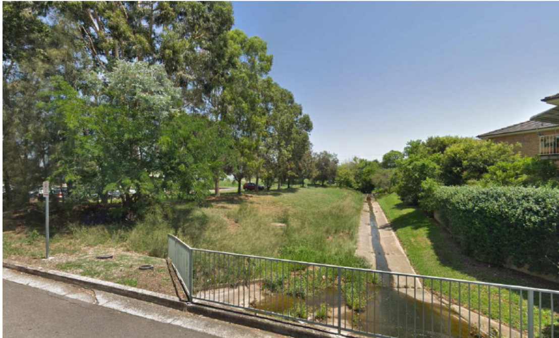
Photograph 1 - looking to the northwest showing the managed vegetation in the watercourse between the carpark and the Mountain View Retreat Retirement Village (on the right).
