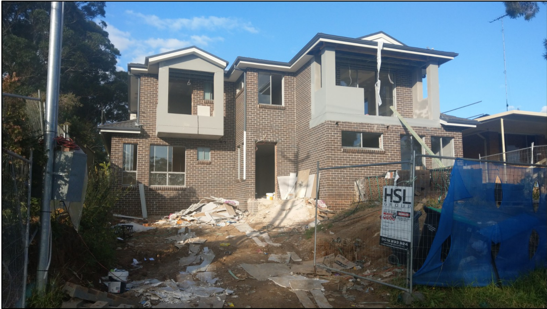
Figure 17: Approved boarding house located at 36 Manning Street currently under construction
