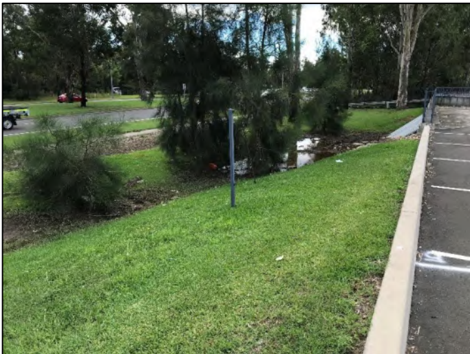
Plate 5 – View towards Forrester Road of stormwater drainage and drainage on the edge of the site.
