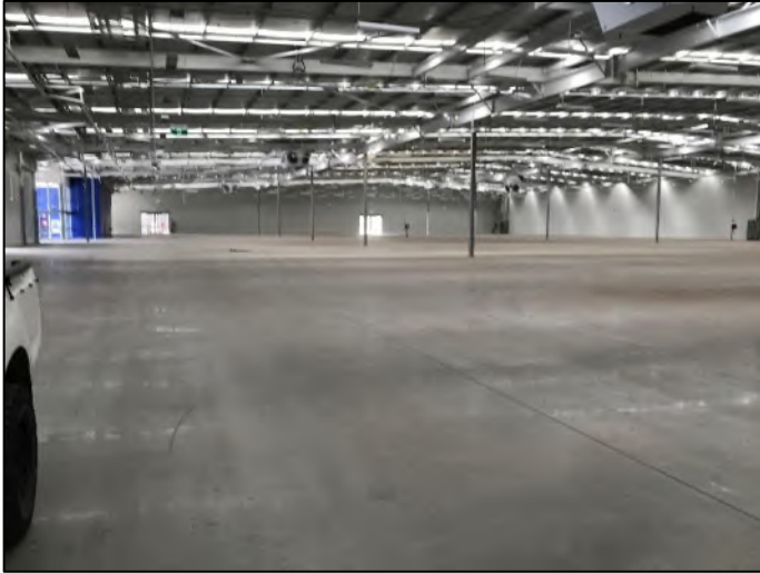
Plate 1 – View north, empty warehouse floor.
