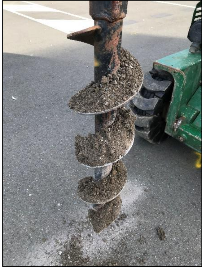
Plate 8 – Road base material encountered.
