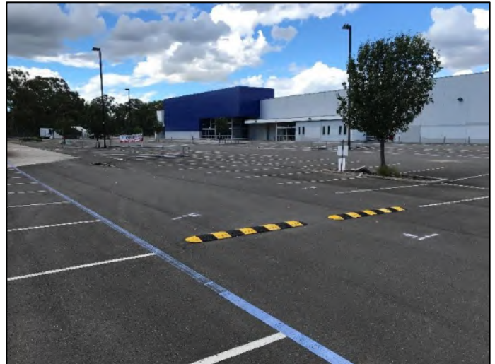
Plate 4 – Looking north-east towards the former bulky goods store.
