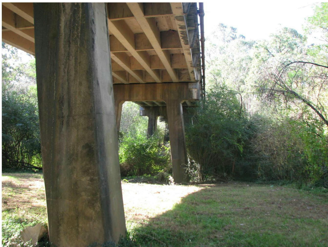
Figure 3 The underside of the South Creek Bridge
