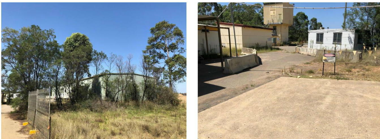
Figure 12 Existing vegetation and hardstand areas are also to be removed
