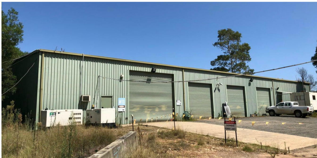
Figure 5 Structure 1, known as 'Kev's Shed'
