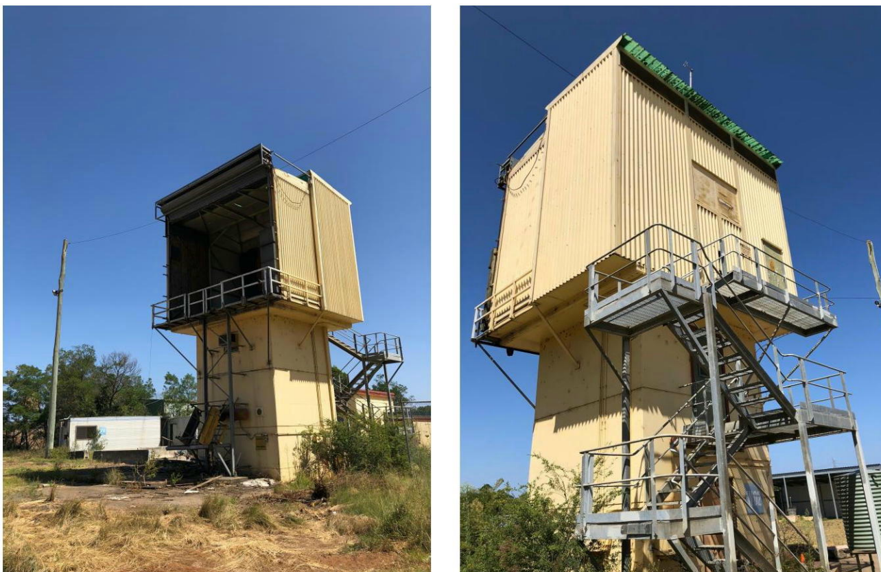
Figure 8 Structure 7 to be demolished and removed
