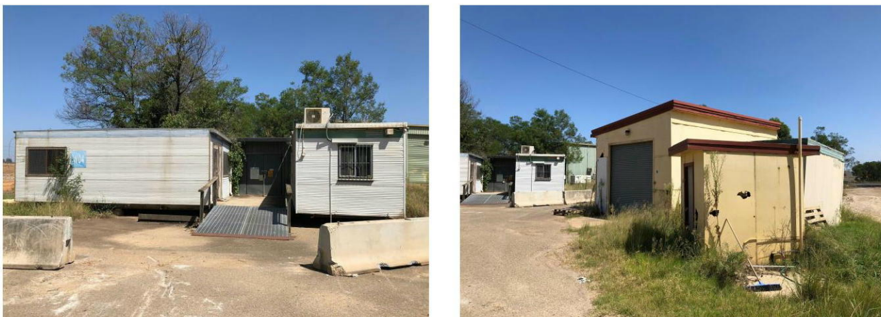
Figure 7 Structures 3, 4 and 5, the temporary veterinary facilities, and Structure 6
