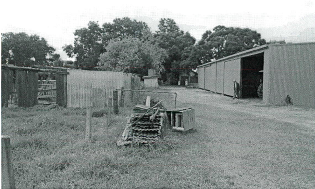
Figure 3: View of site from north
