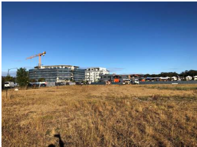
Photo 3: Construction occurring in the area, apartments are present to the south west
