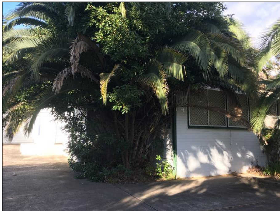
Figure 12: The front elevation of the building, including a view of Tree 21 (Canary Island Date Palm).
