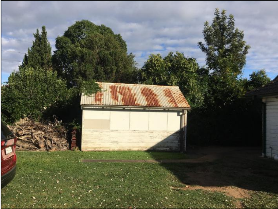
Figure 15: Shed at the rear of the site.
