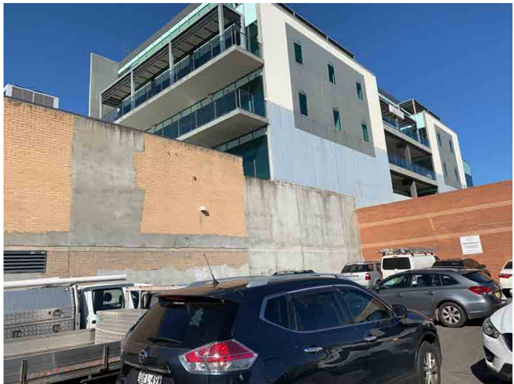
Asphalted car park fronting Lawson Lane to the rear of the primary site view to south.
