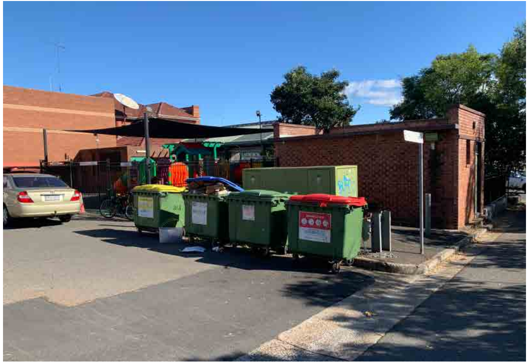
View west of the subject site substation and playground from Lawson Lane
