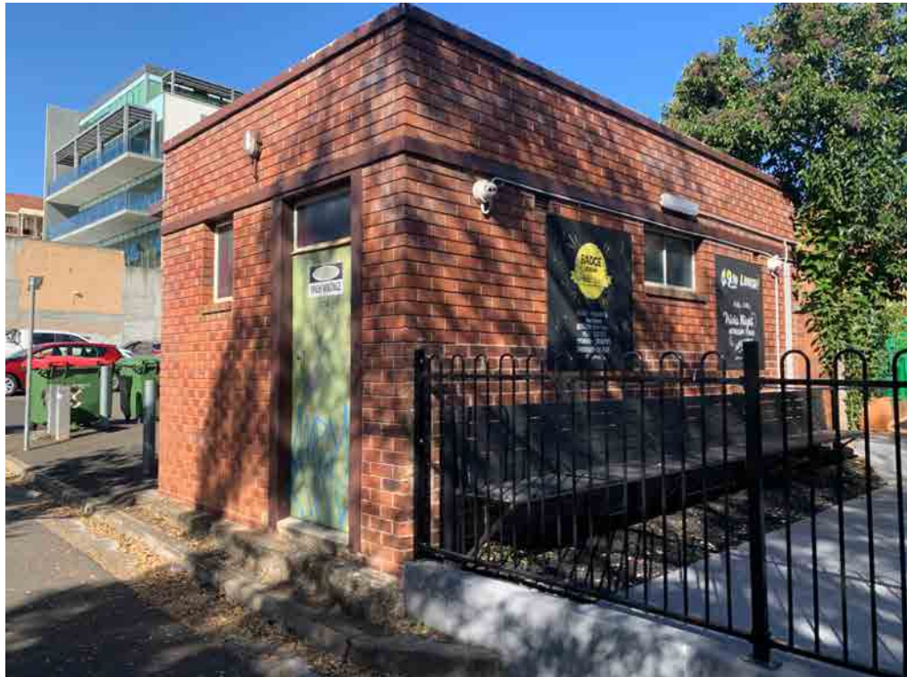
View of the substation from Lawson Lane
