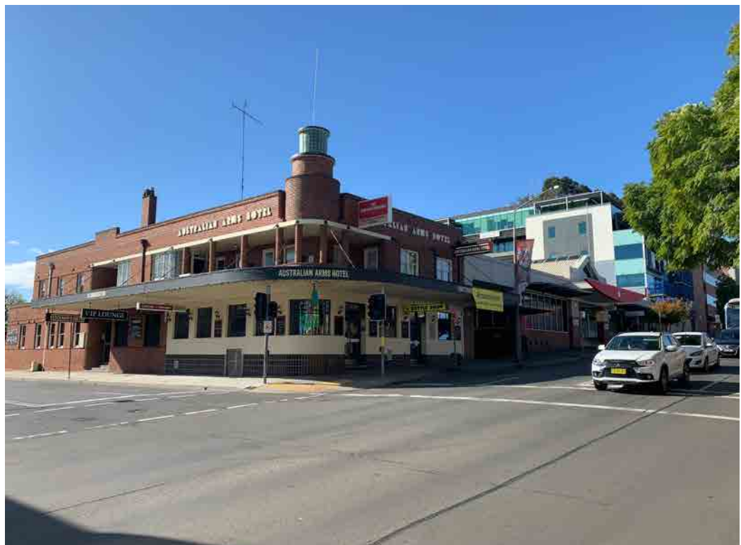
Australian Arms Hotel view towards north-east High Street and Lawson Street
