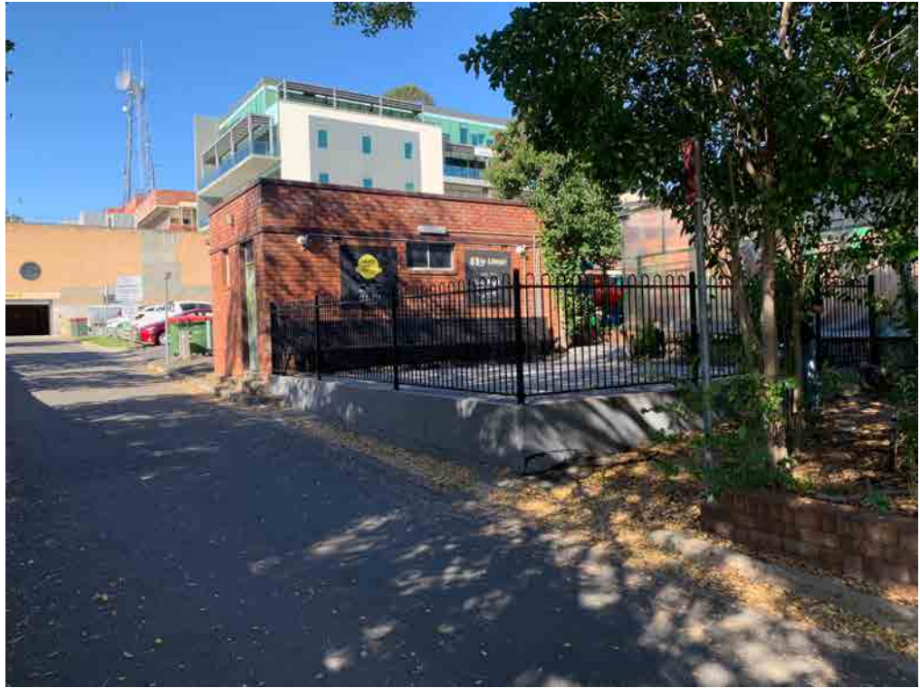
View east of the subject site substation and playground from Lawson Lane
