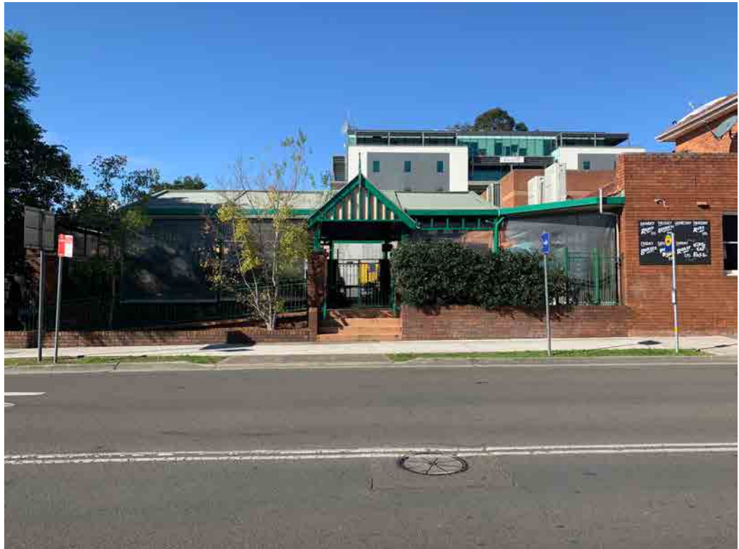
Covered beer garden on north-west of the site
