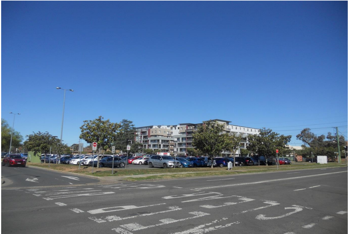
Figure 15 View South Towards Nearby Council Owned Car Park – Intersection of Union Lane and Worth Street
