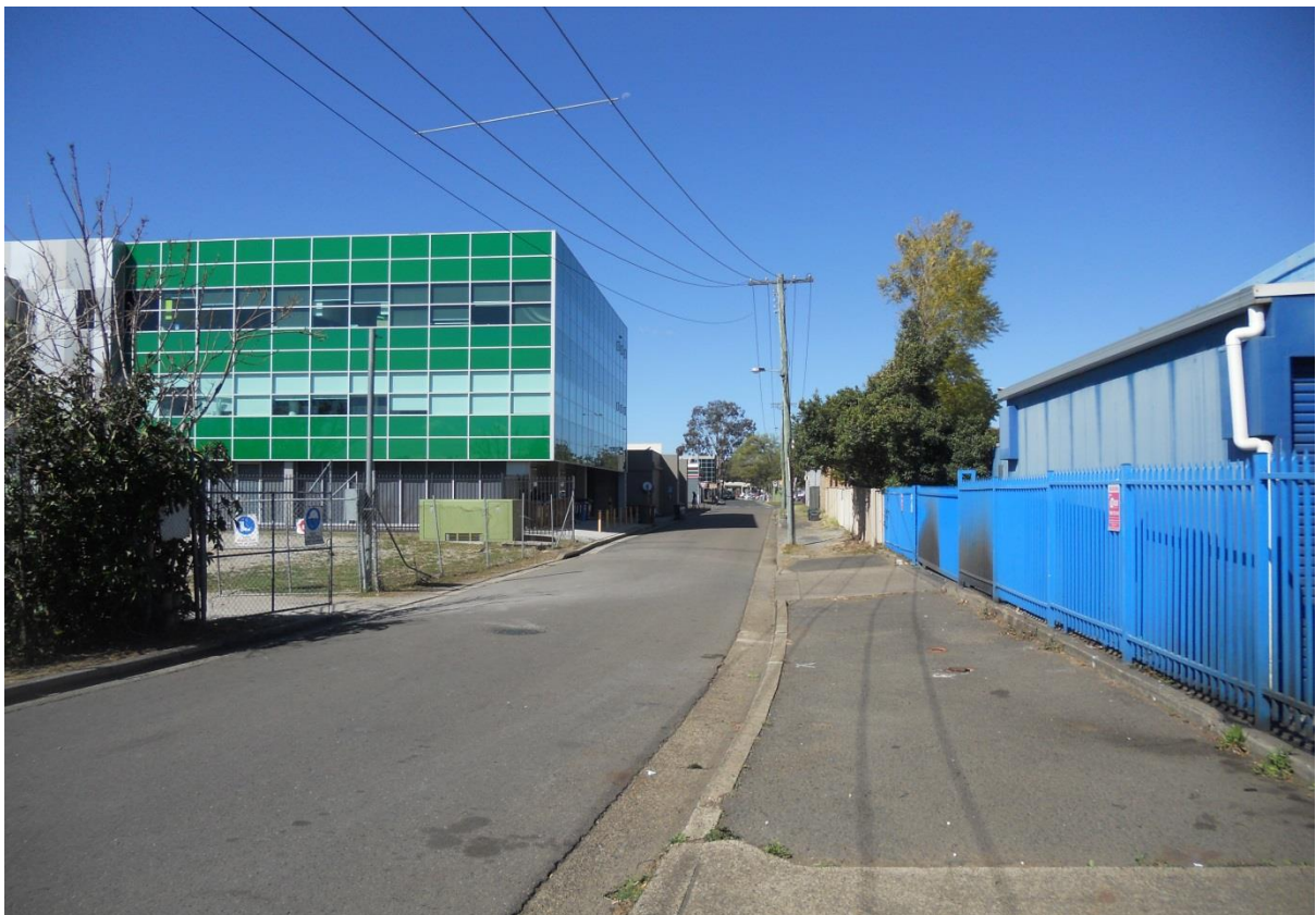
Figure 8 View East Along Streetscape of Union Lane
