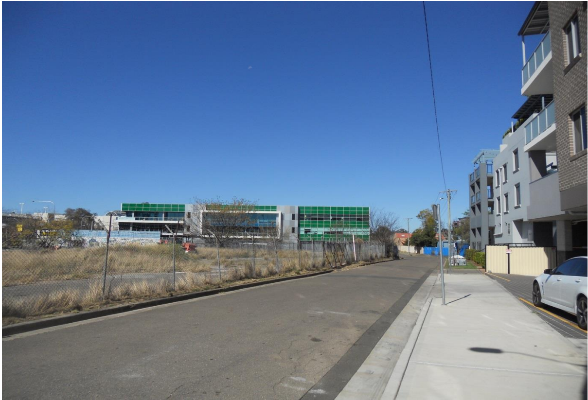
Figure 9 View East Along Streetscape of Union Lane
