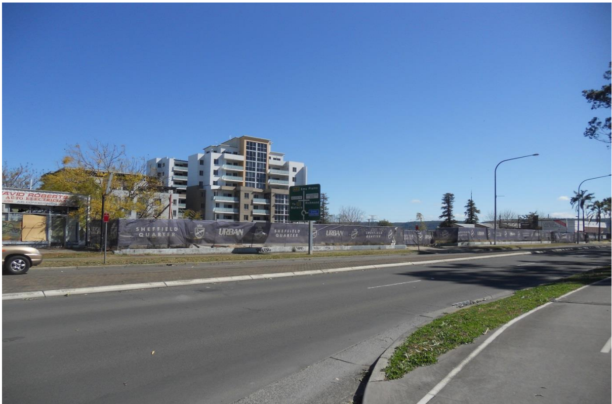
Figure 10 View South-West Towards Adjoining Vacant Site - 614 High Street
