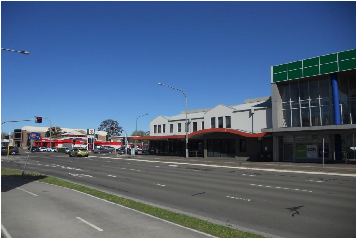
Figure 14 View South- East Towards Adjoining Low to Medium Rize Commercial Buildings
