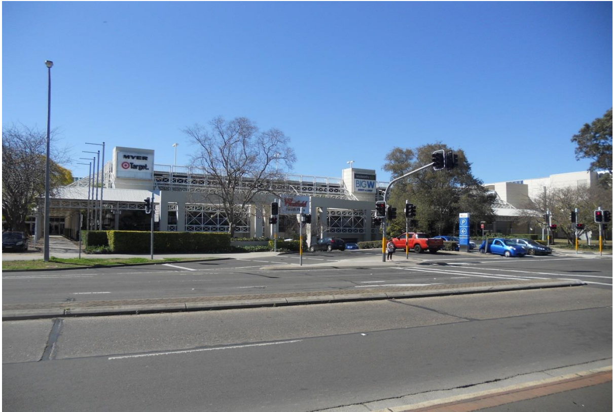
Figure 11 View North Towards Westfield Shopping Centre
