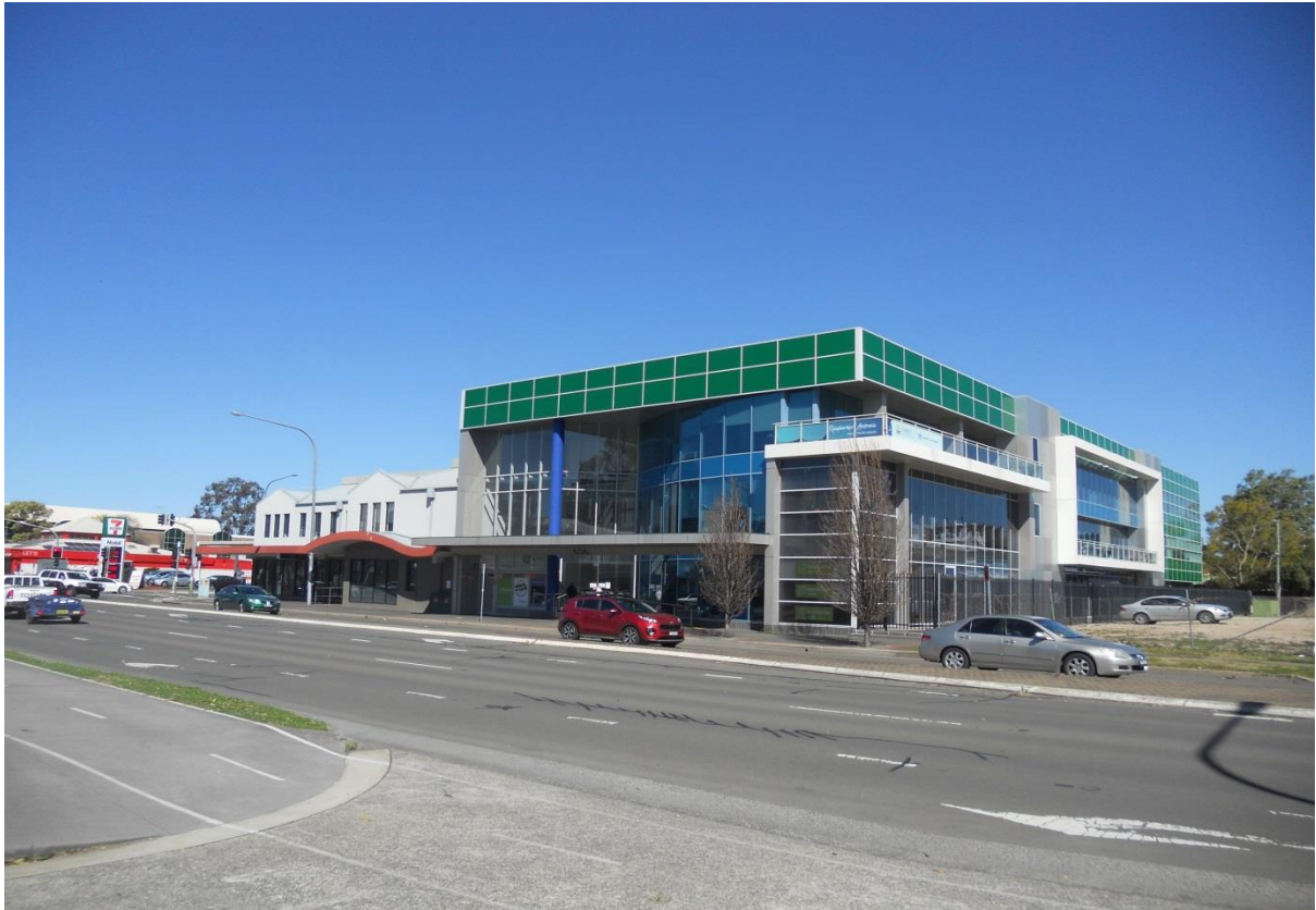
Figure 5 View South Towards Commercial Buildings - 604 - 606 High Street
