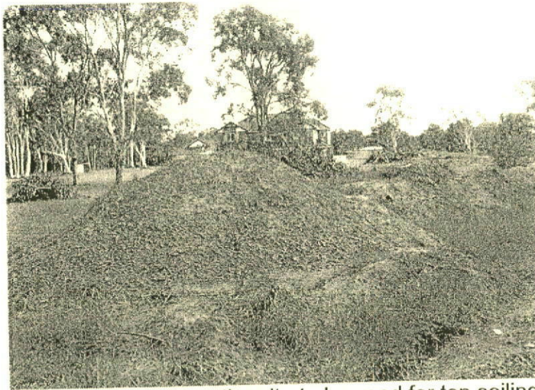
Natural excavated material from the site to be used for top soiling of property
