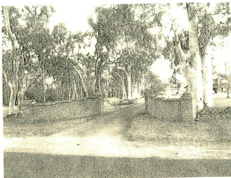
Existing front feature entry fence
