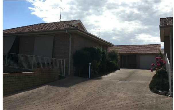
Figure 11 No. 68 Doonmore Street
