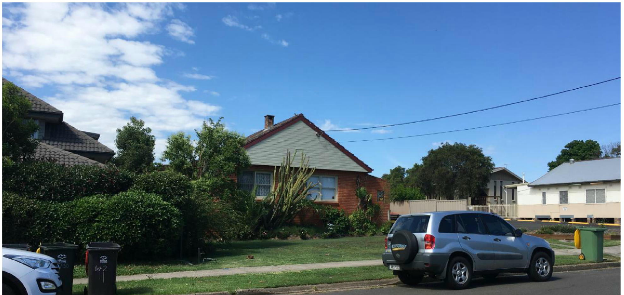
Figure 3 No. 154 Stafford Street
