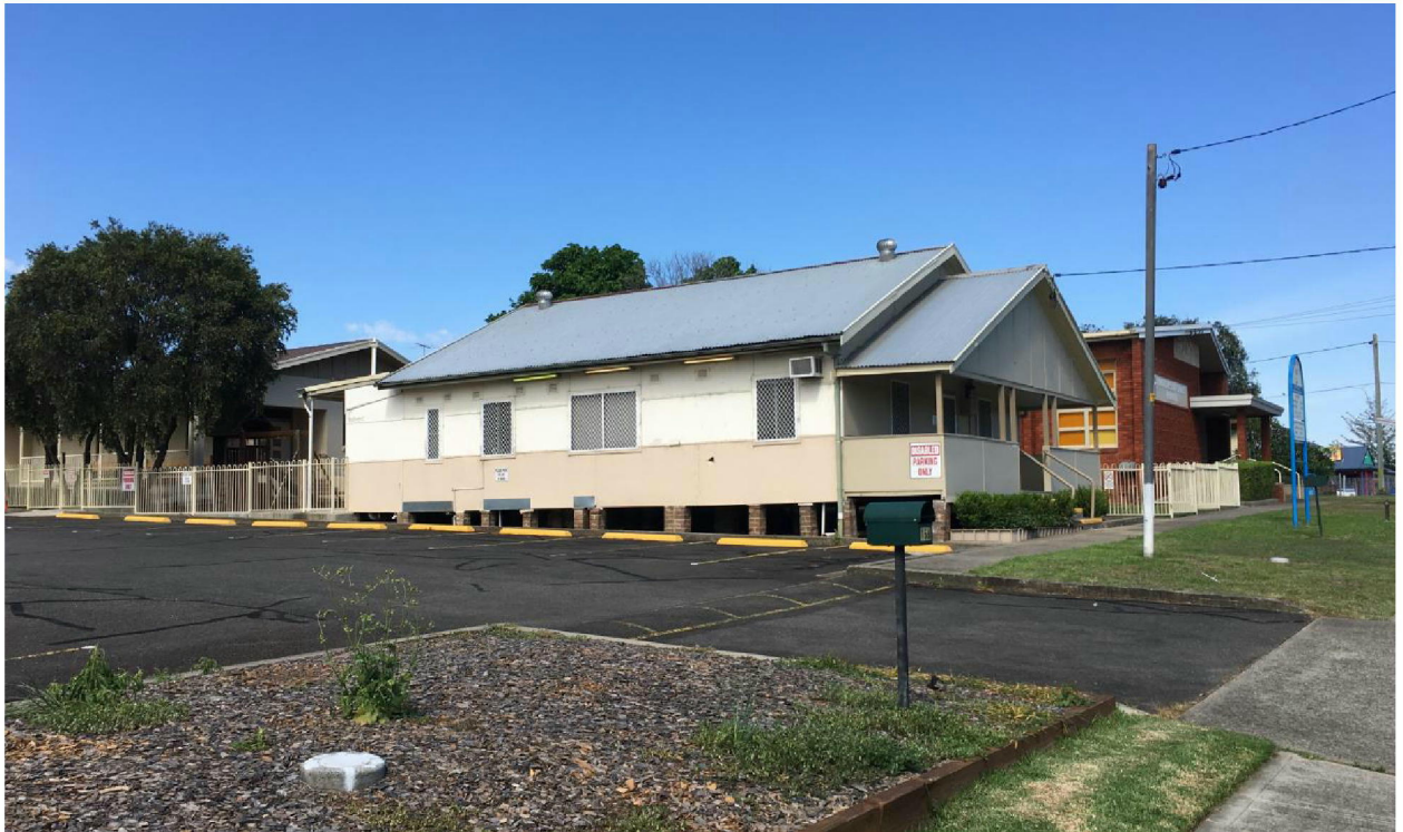
Figure 2 Existing Church of Christ administration building (front) and church (face brick building behind) located at No. 156-160 Stafford Street.
