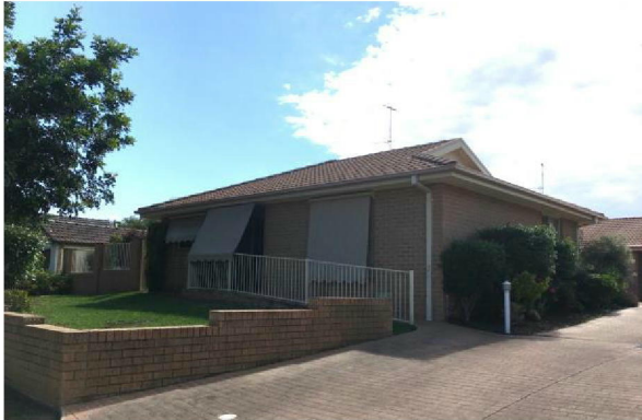
Figure 10 No. 68 Doonmore Street
