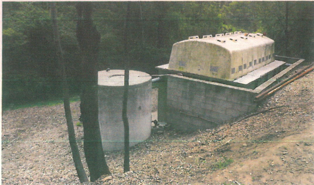
View of existing sewerage treatment plant, adding a suitable bund wall to collect any overflow or spillage can easily be accommodated.
