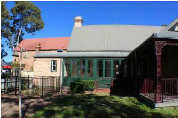
Photo 3: The enclosed verandah at the rear of the building
