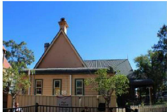
Photo 4: The rear façade of the building
