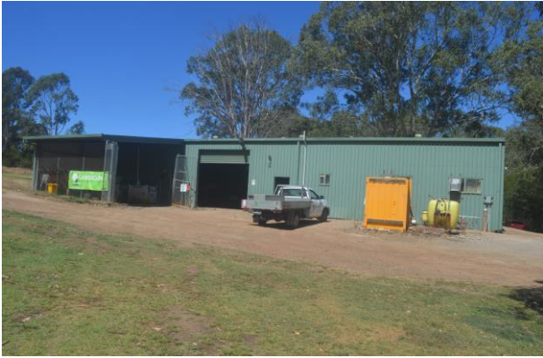
Picture 3 – Maintenance shed
