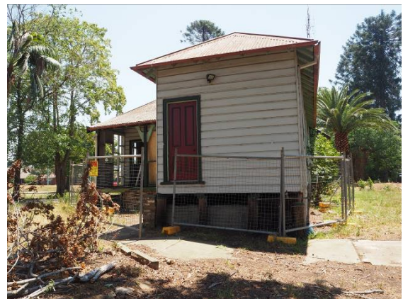
Figure 7: Southern (rear) elevation of former Police Station Building and location of proposed extension.
