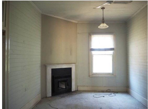
Figure 13: Interior view of existing living room (room 5), looking east.
