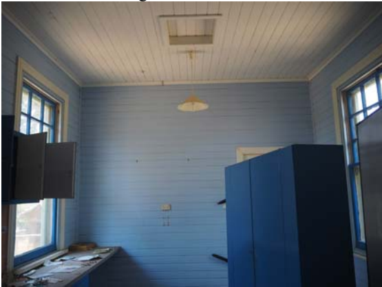
Figure 12: Interior view of existing kitchen looking south (room 8).
