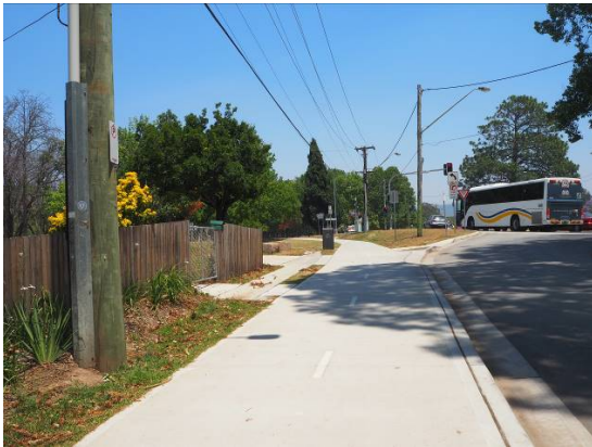
Figure 4: Punt Road, looking west towards the Great Western Highway. The front (north) fence boundary of 4 Punt Road is to the left of frame.
