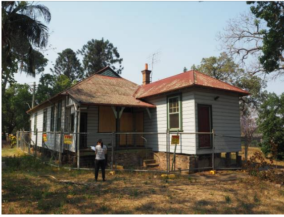
Figure 8: Southern (rear) elevation of former Police Station Building.
