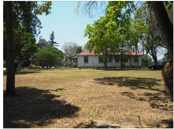
Figure 5: Western elevation of the former Police Station Residence, looking across the adjacent allotment.
