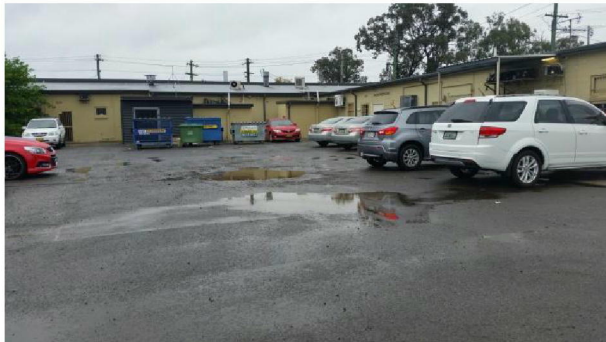
Photo 2: Rear view, looking south
