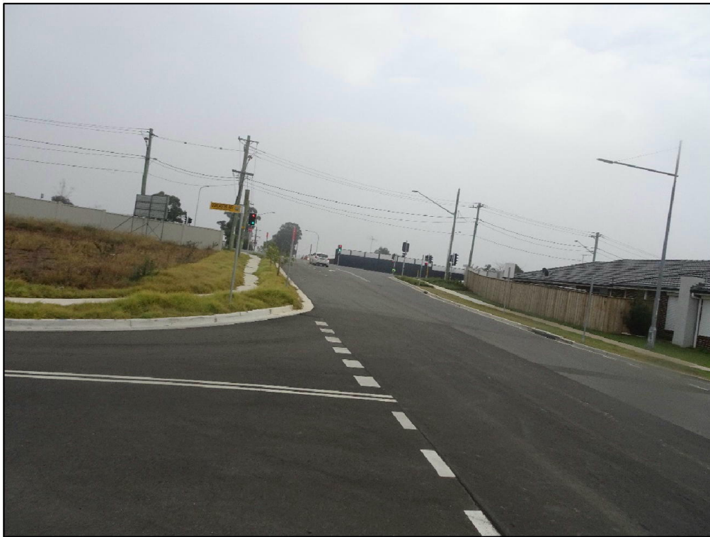
Figure 4b: Caddens Road looking West from adjacent to Doncaster Avenue
