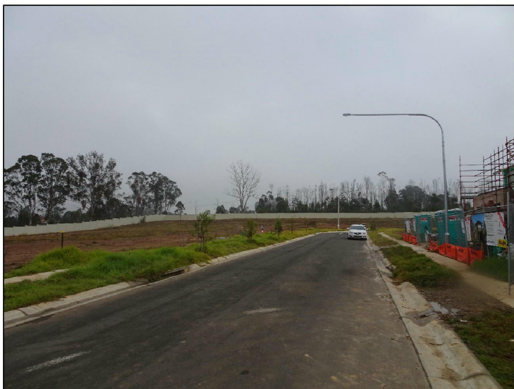
Figure 4a: Doncaster Avenue looking West near looking towards childcare site
