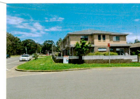
Boarding house at 2 Edward Street, Kingswood
