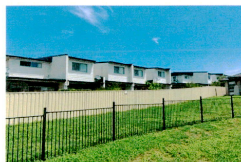
Rear of townhouses at 76 Jones Street, Kingswood
