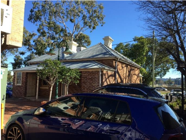
Figure 5 – Rear (north east) elevation, 148 Station Street.
