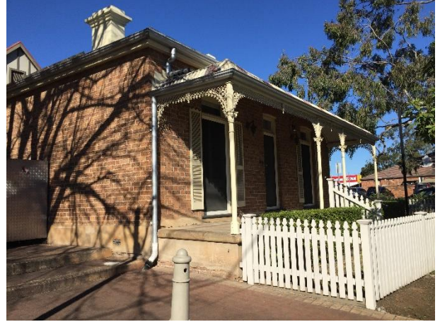
Figure 10 – Front (west) elevation of 148 Station Street looking north to south. Front garden with picket fence. Source: Urbis, July 2019
