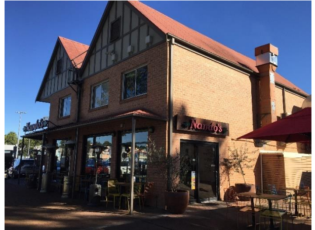
Figure 6 – New building to east of 148 Station Street, occupied at ground floor by Nando's
