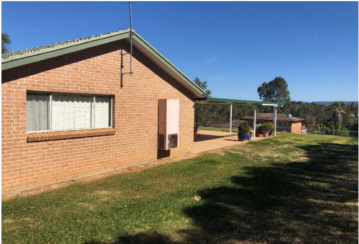
Existing single storey residential dwelling
