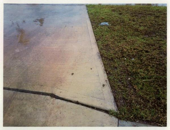
Figure 107 Surface imperfections to pram ramp wing.
