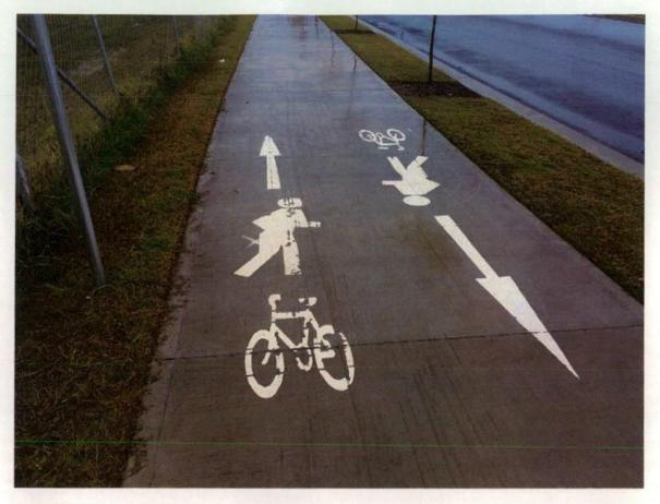
Figure 17 Damage to shared cycleway line marking.
