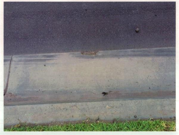
Figure 358 Damage to gutter lip.
