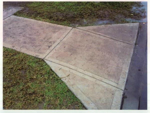
Figure 160 Stains on footpath surface.
