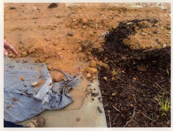
Figure 496 Possible damage to footpath beneath crushed sandstone.
