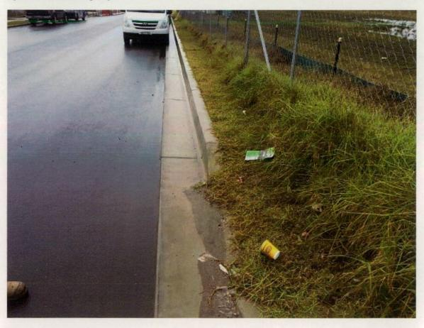
Figure 174 Existing silt in K&G.
