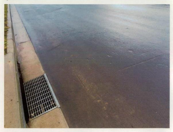
Figure 210 Surface marks and gouges in asphalt.
