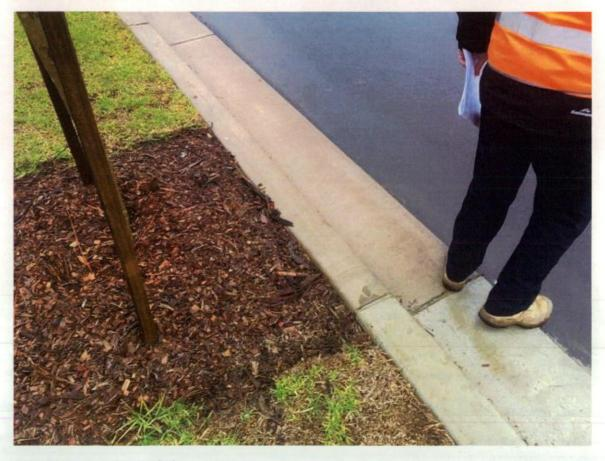
Figure 30 Concrete splatter on kerb.
