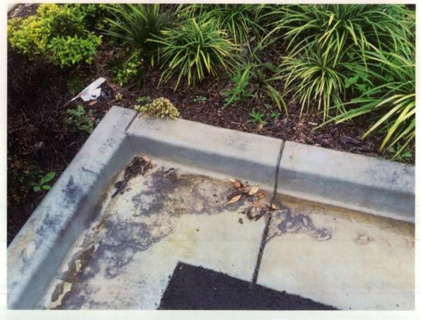
Figure 58 Bitumen stains and tyre marks on kerb.
