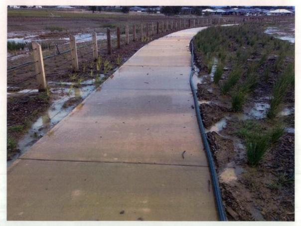
Figure 462 Holding water in wheel ruts.
