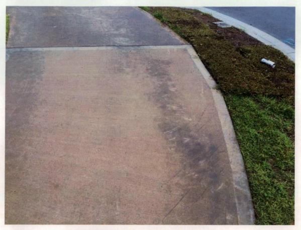
Figure 241 Tyre marks on pavement.
