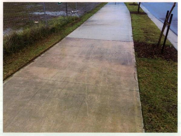
Figure 22 Scratches and marks to pavement surface.
