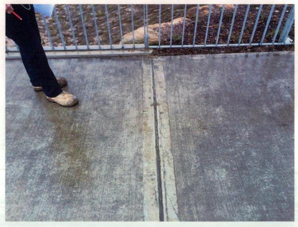
Figure 10 surface damage to concrete footpath and staining.
