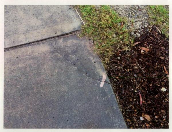
Figure 336 Crack in concrete footpath.
