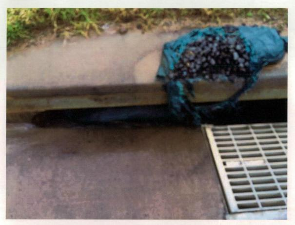
Figure 409 Existing silt control, breaking up and going down the drain.
