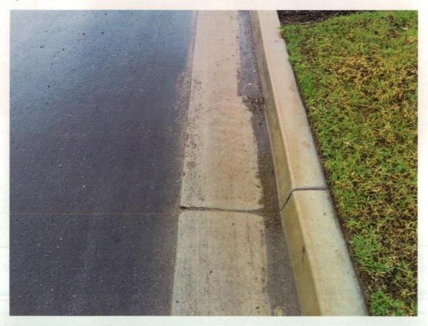
Figure 267 Surface imperfections on gutter.
