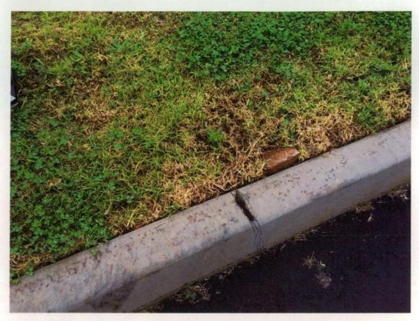
Figure 65 Large crack at kerb joint.
