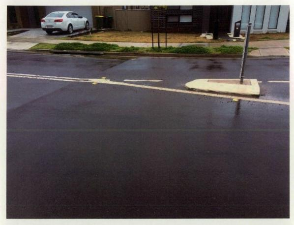
Figure 123 Line marking damaged.
