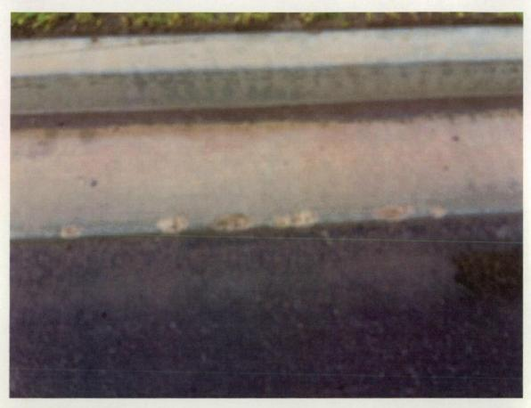
Figure 249 Damage to gutter lip.
