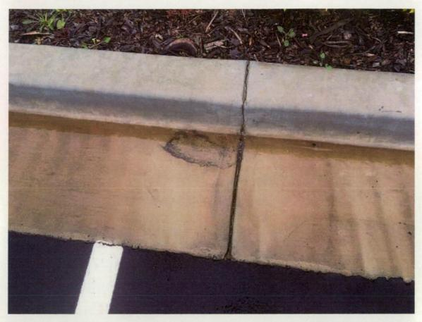
Figure 63 Wide crack in joint.
