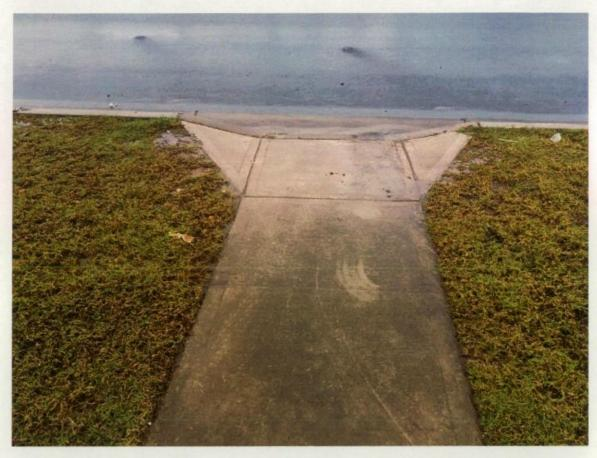
Figure 149 Damage to footpath surface.
