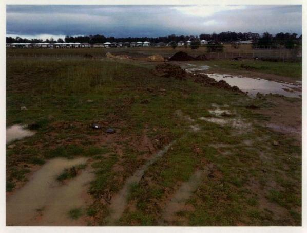
Figure 444 Wheel ruts and soil untidy in areas, holding water.
