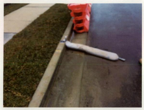
Figure 403 Existing silt controls.
