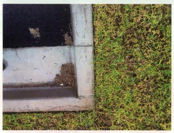
Figure 85 Crack in kerb.
