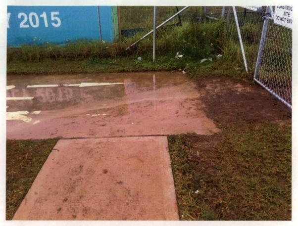
Figure 163 Erosion and soil egress from site.
