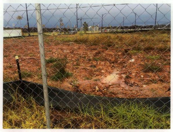
Figure 125 Subgrade holding water.
