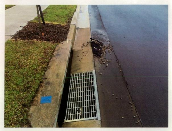
Figure 419 Existing silt controls broken and going down drain.
