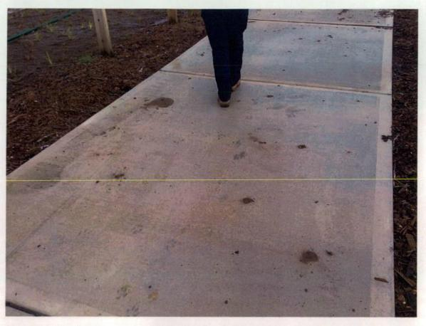
Figure 517 marks on footpath surface.
