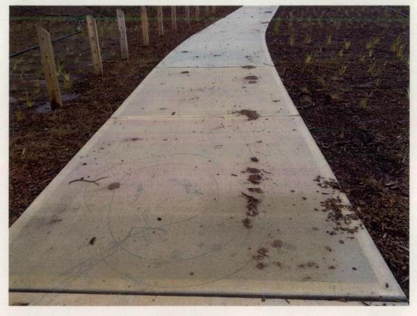
Figure 520 Scratch marks and excess soil on footpath surface.
