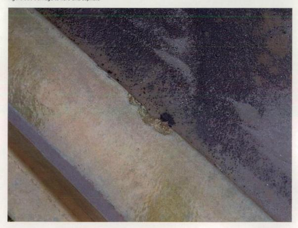
Figure 317 Gutter lip damaged.
