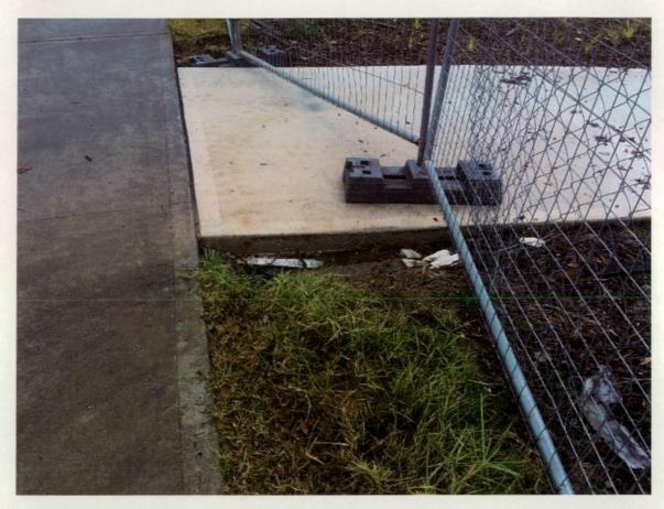
Figure 379 Soil low and holding water near to footpath.
