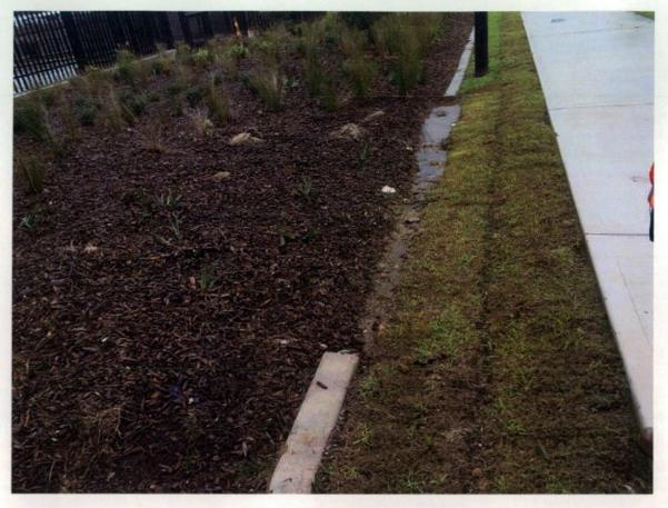
Figure 361 Concrete edge incomplete and holding water.
