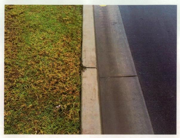
Figure 135 Chips to back of kerb.
