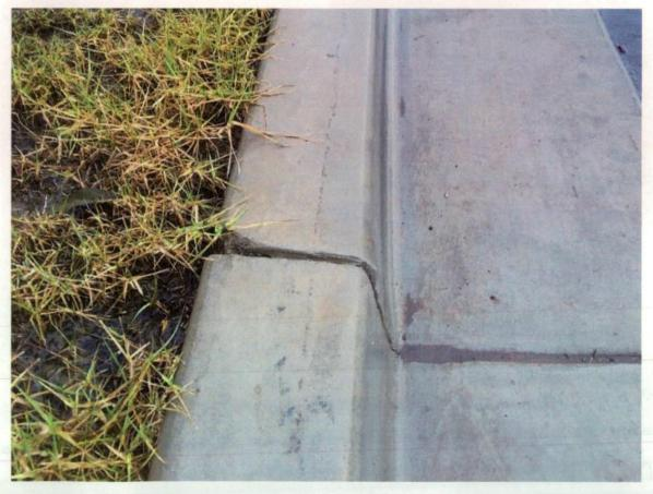
Figure 224 Damage at kerb joint.
