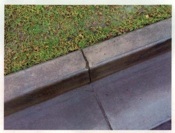
Figure 159 Damage on kerb joint.
