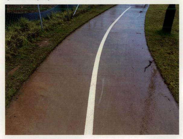
Figure 124 Line marking damaged.
