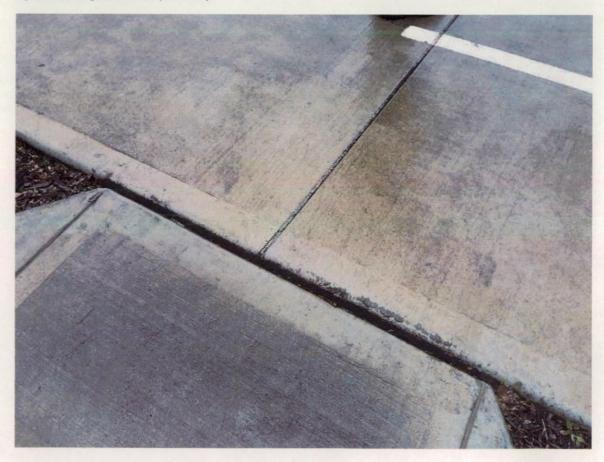
Figure 92 Concrete splatter on footpath.
