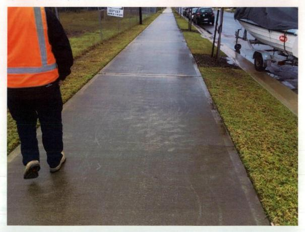
Figure 315 Tyre marks on footpath.
