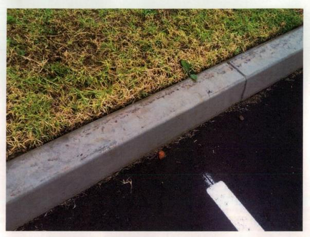
Figure 77 Staining and surface cracking to kerb.
