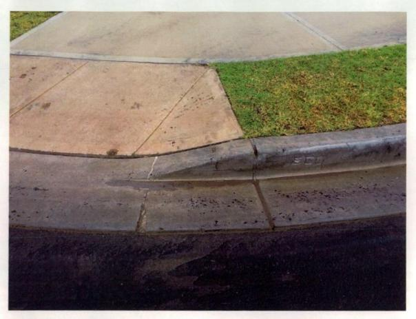
Figure 237 Bitumen stains on pram ramp and K&G.
