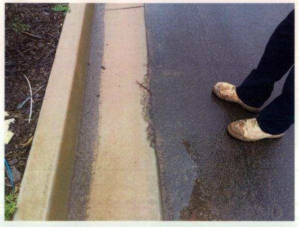
Figure 295 Damage to gutter lip.
