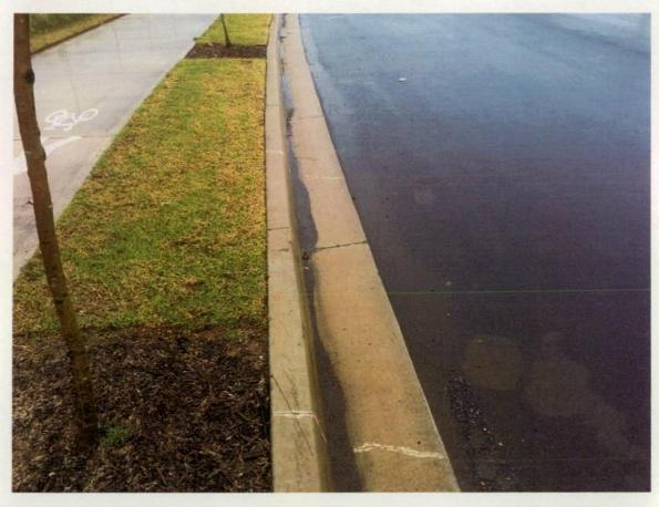
Figure 15 Cracks repaired in K&G.
