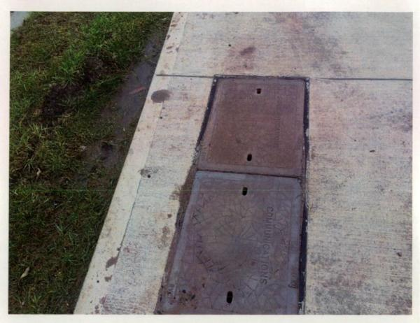
Figure 344 Damage around Telstra pits and concrete splatter.
