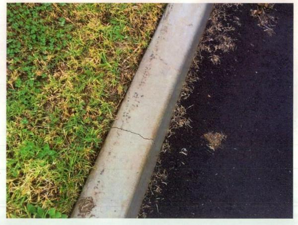
Figure 74 Surface cracks to kerb.
