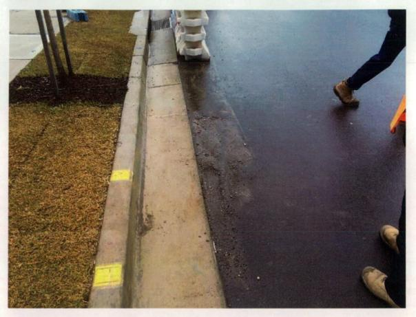
Figure 401 damage to asphalt, repaired crack in K&G.
