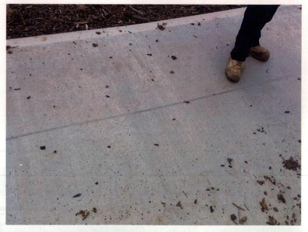
Figure 534 Scratches on footpath surface.
