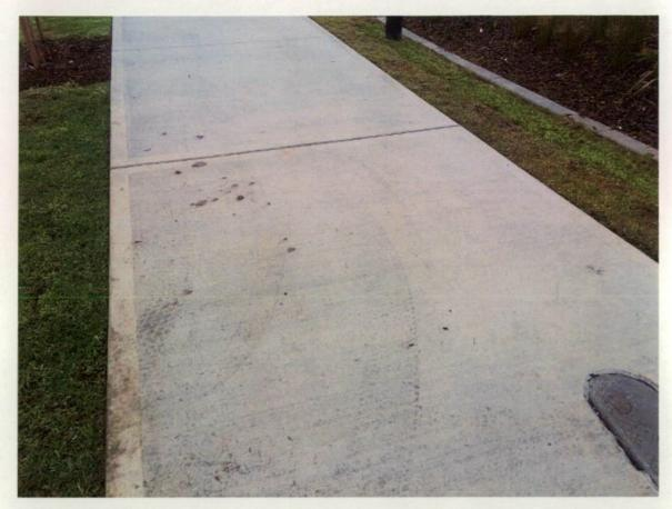
Figure 363 Marks on concrete footpath.
