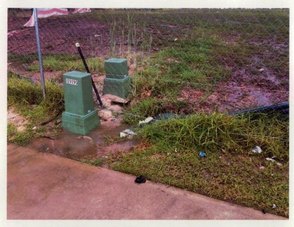
Figure 137 Subgrade and sand erosion, silt controls failing.
