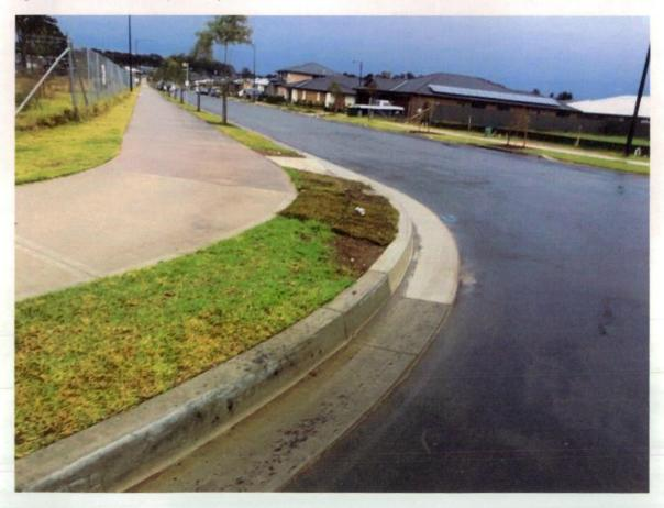
Figure 238 Bitumen stains on pram ramp and K&G, turf missing.
