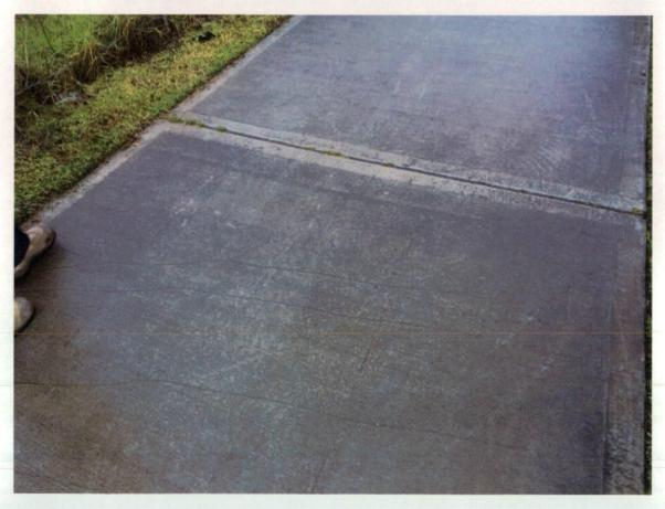
Figure 263 Scratches on concrete surface.
