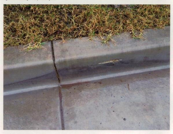
Figure 218 Gouge to face of kerb.
