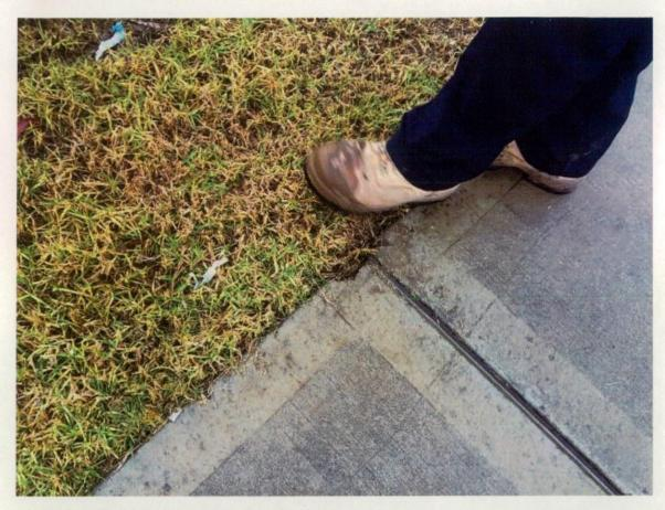
Figure 280 Damage to edge of footpath.
