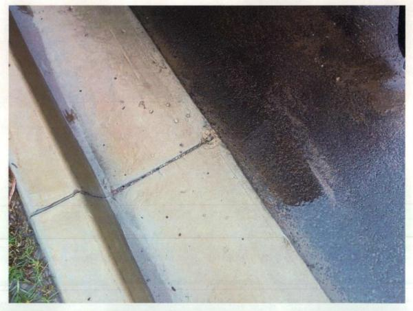
Figure 319 Damage on concrete joint.
