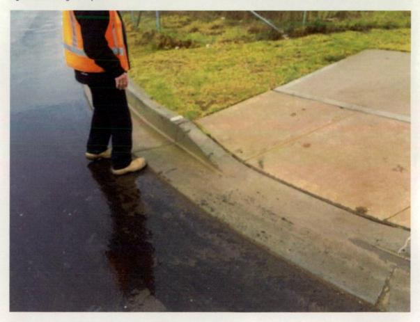
Figure 236 Bitumen stains on pram ramp and K&G.
