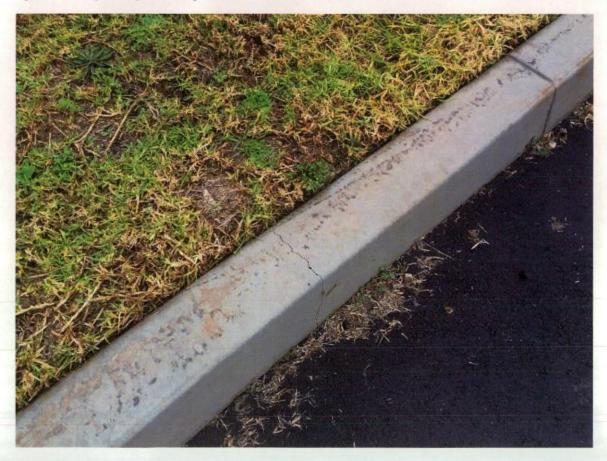
Figure 78 Cracks in concrete kerb.
