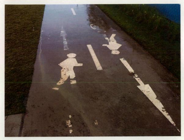
Figure 165 Damage to cycleway line marking, soil egress.
