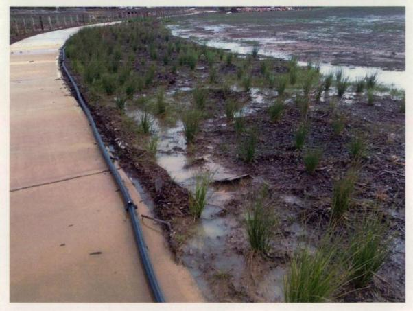
Figure 464 Water runoff through garden, holding water.
