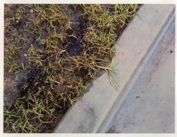
Figure 221 Damage to back of kerb.
