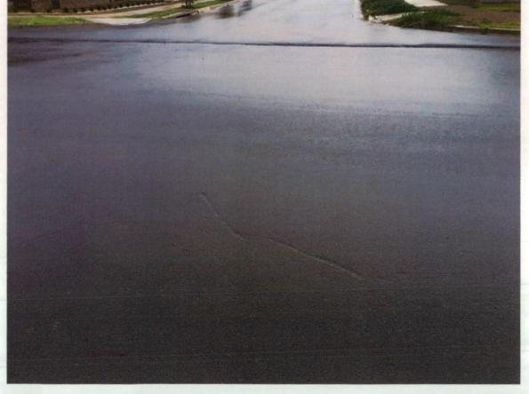
Figure 176 Gouge in existing asphalt.
