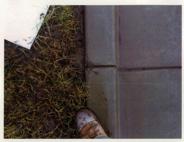
Figure 228 Damage on back of kerb.
