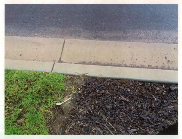
Figure 252 Damage to back of kerb.
