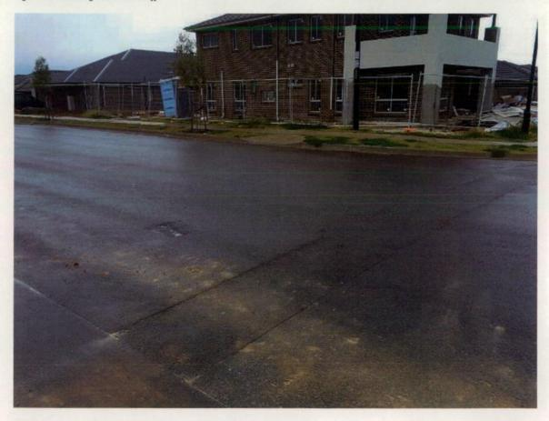
Figure 392 damage to asphalt and silt runoff from sites opp. Oval.
