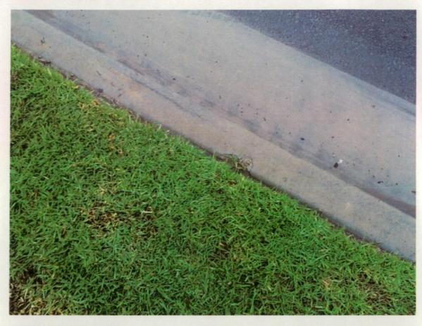
Figure 359 Damage to gutter lip.
