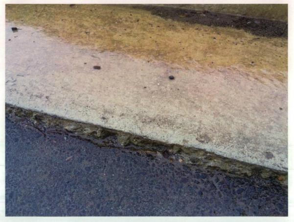
Figure 14 Damage to gutter edge.
