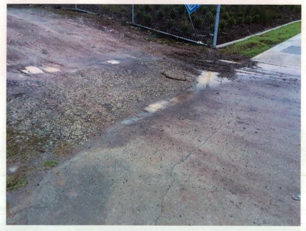
Figure 339 Crack in concrete footpath.
