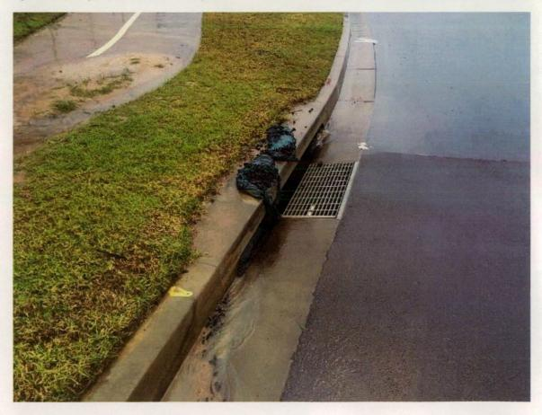
Figure 120 Existing sediment controls in disrepair.
