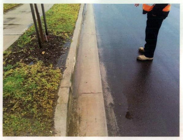
Figure 381 Concrete stains on asphalt.
