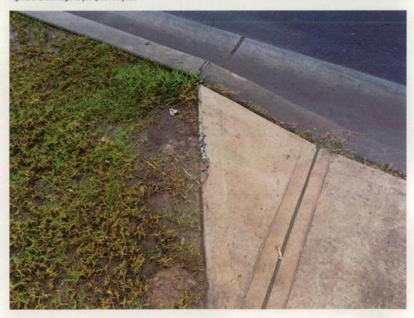
Figure 150 Damage to pram ramp wing.
