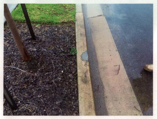
Figure 290 Concrete patching.
