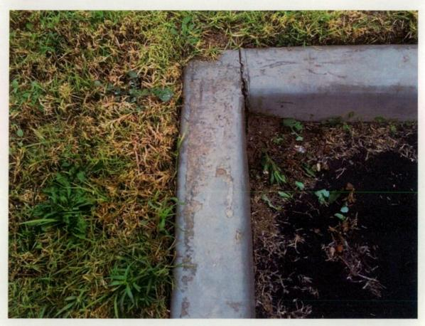
Figure 75 Stains and chips on top of kerb.
