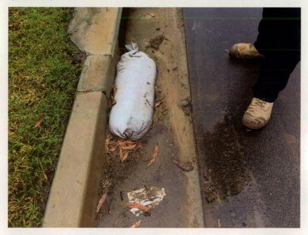
Figure 321 Existing sediment controls full of silt.
