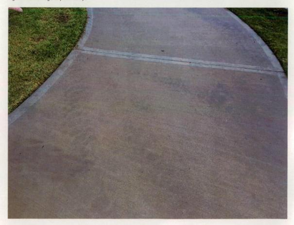
Figure 240 Tyre marks on pavement.
