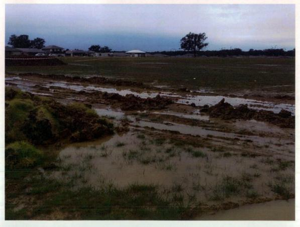
Figure 438 Wheel ruts holding water.
