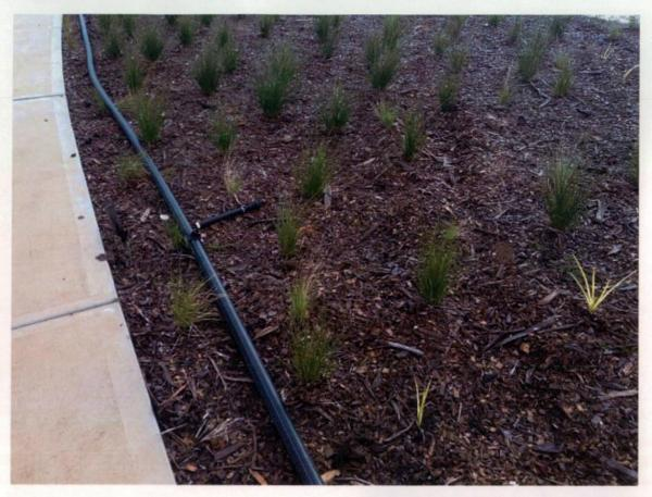
Figure 473 Broken irrigation, wheel ruts in garden.
