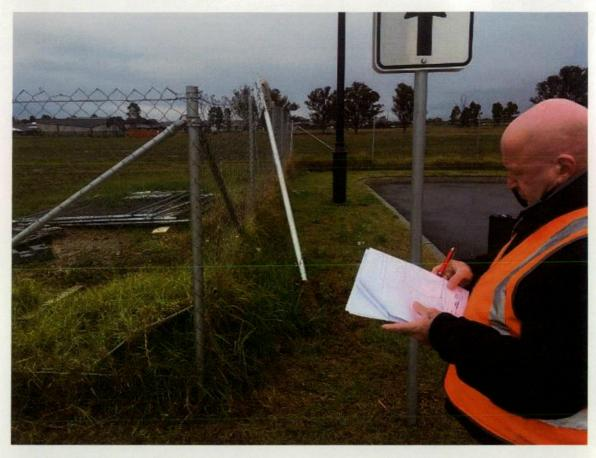
Figure 35 Sign knocked out of foundation.
