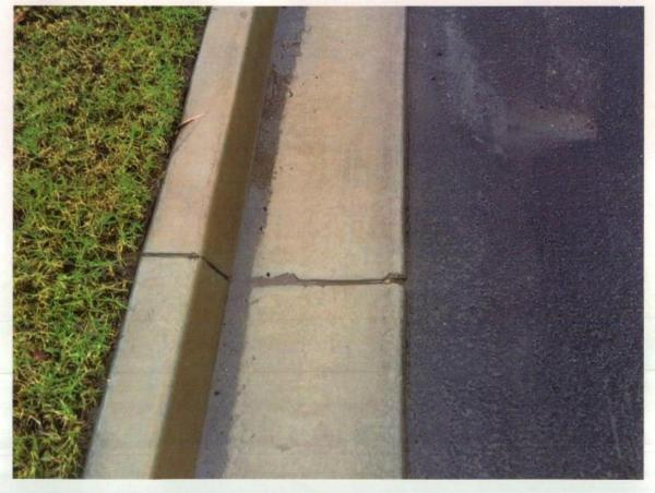
Figure 303 Damage at concrete joint.
