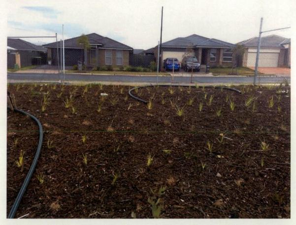
Figure 527 Excess irrigation material left on site.
