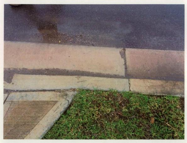
Figure 292 Damage to pram ramp and kerb.
