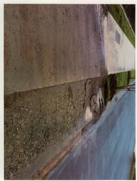
Figure 340 Crack in concrete footpath.
