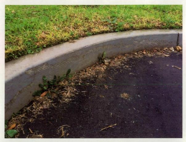
Figure 47 Damage to kerb.
