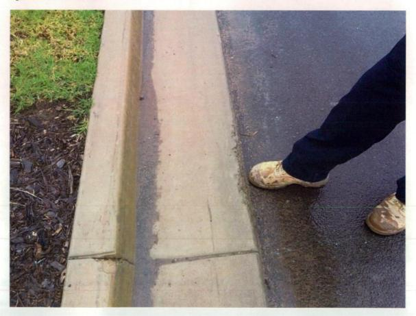
Figure 275 Damage to joint and gutter lip.
