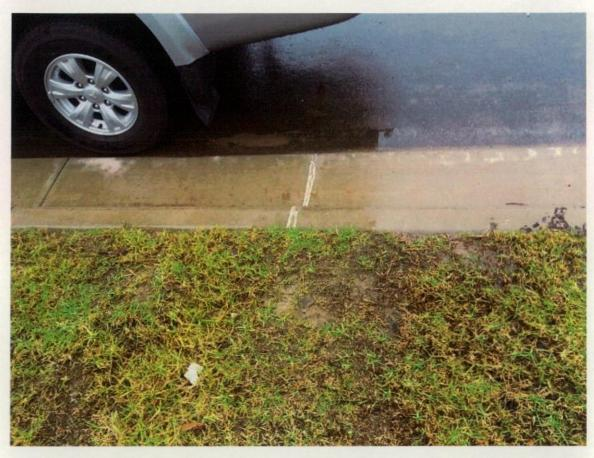
Figure 332 previously repaired concrete crack in K&G.
