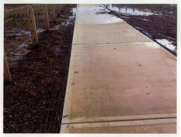
Figure 485 Cables cut from handrail near riparian
