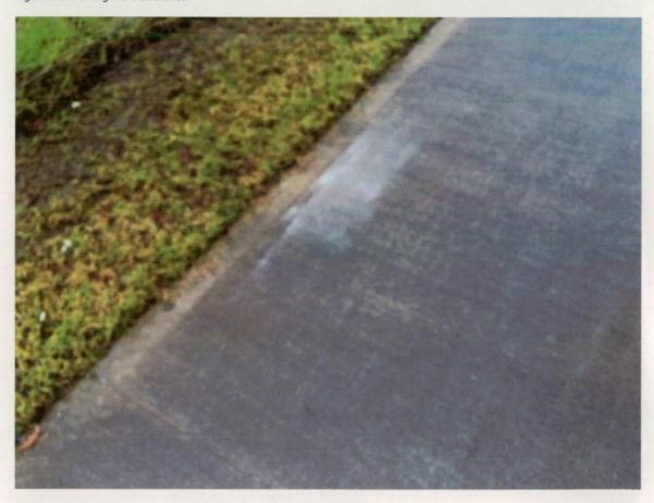
Figure 313 Surface damage to footpath.
