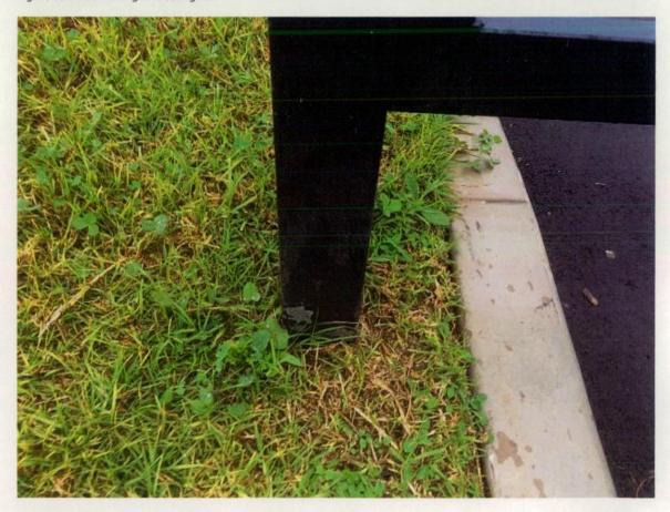
Figure 40 Paint missing on boom gate.
