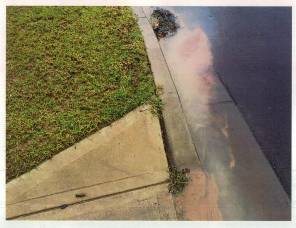
Figure 122 Surface marks to pram ramp, holding water.
