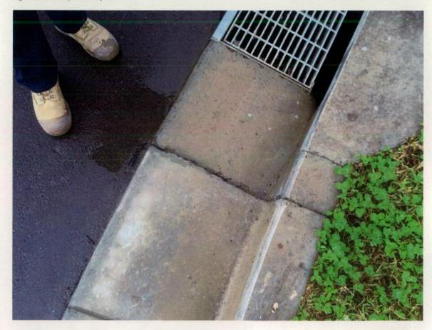
Figure 396 Large height difference between lintel and gutter.
