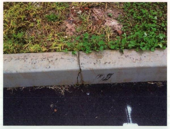
Figure 82 Crack in kerb.
