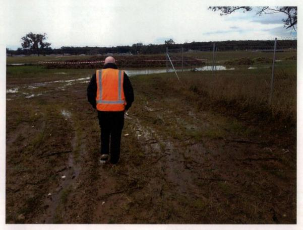
Figure 429Holding water in wheel ruts.
