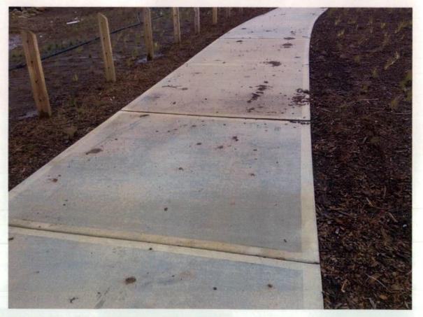
Figure 518 Scratches and excess soil on footpath surface.
