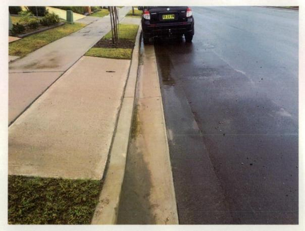
Figure 383 silt runoff in gutter.
