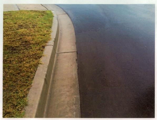
Figure 233 Damage to gutter lip.
