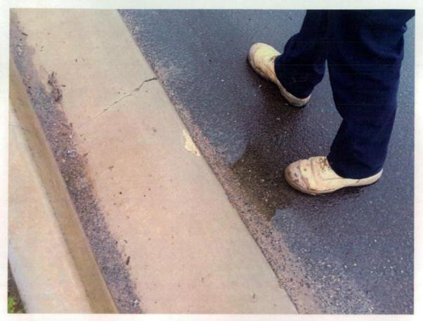
Figure 258 Patch on gutter lip.
