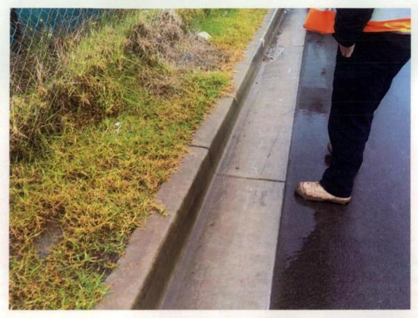
Figure 171 concrete splatter on kerb.
