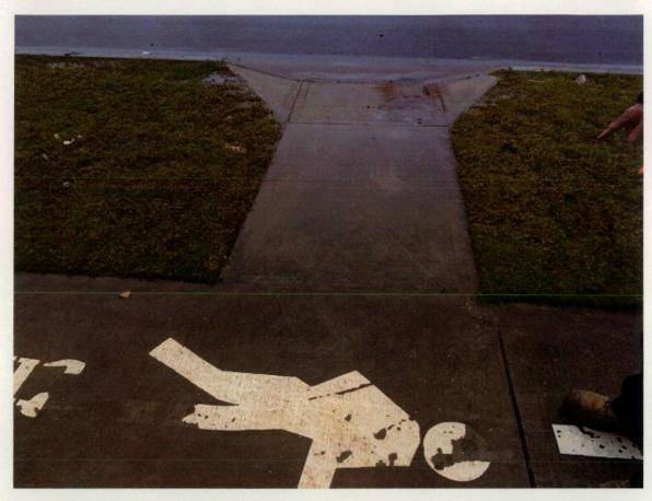
Figure 157 Surface damage to concrete footpath.
