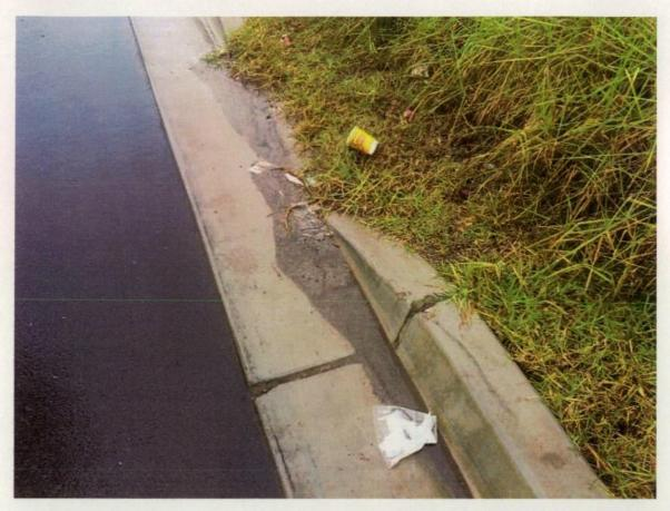
Figure 173 Silt and damage to joint.
