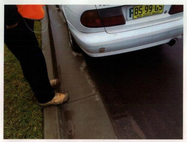
Figure 330 Patching to lip of gutter.
