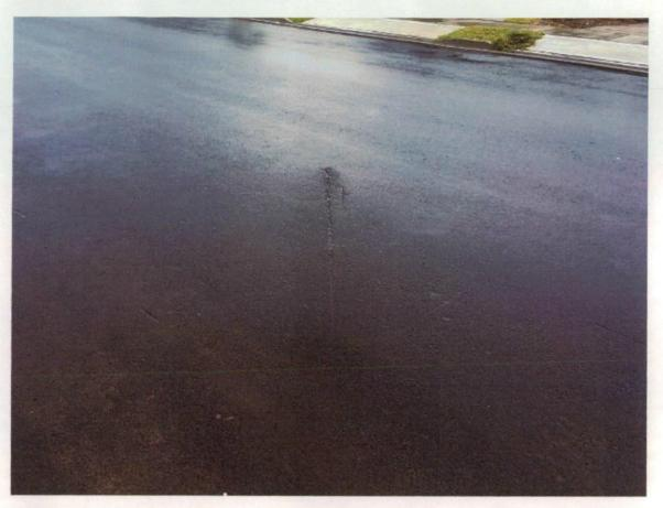
Figure 215 Gouge in asphalt.
