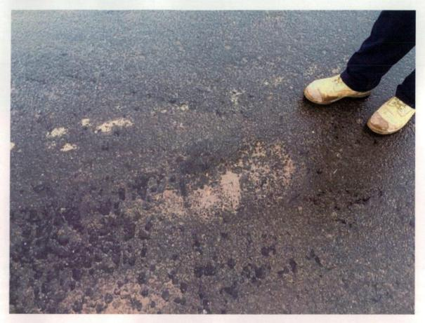
Figure 393 Surface damage to asphalt.
