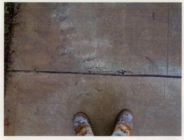
Figure 142 Machinery damage to footpath.
