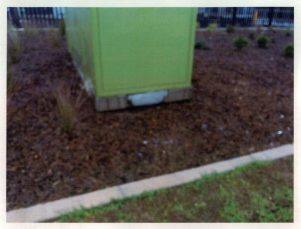
Figure 357 Mulch has been washed out from under electrical box.
