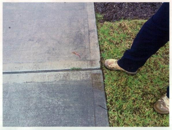
Figure 279 Damage to edge of footpath.
