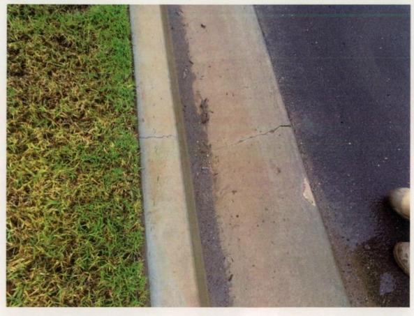
Figure 257 Crack in kerb.
