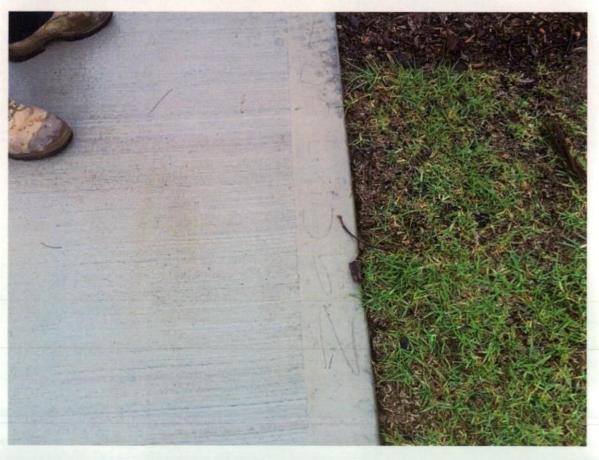
Figure 26 Writing scratched into concrete footpath.
