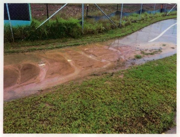
Figure 121 Footpath holding water and silt.
