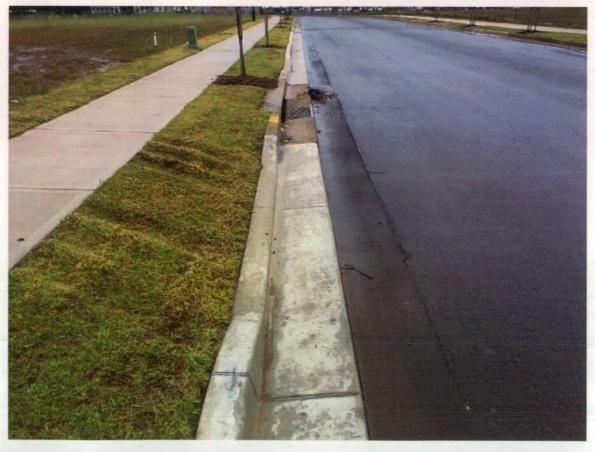
Figure 418 Marks on K&G, wheel ruts in turf area.
