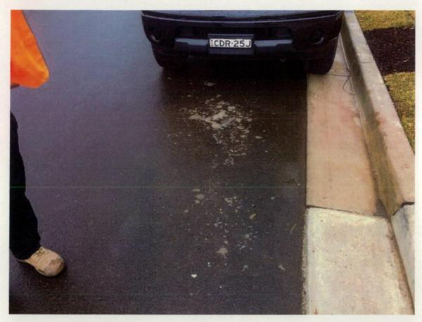
Figure 399 Concrete splatter on asphalt.
