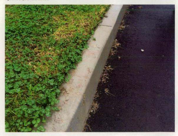
Figure 72 concrete splatter to top of kerb.
