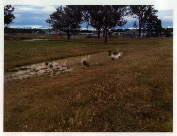
Figure 421 Site holding water in low spot.
