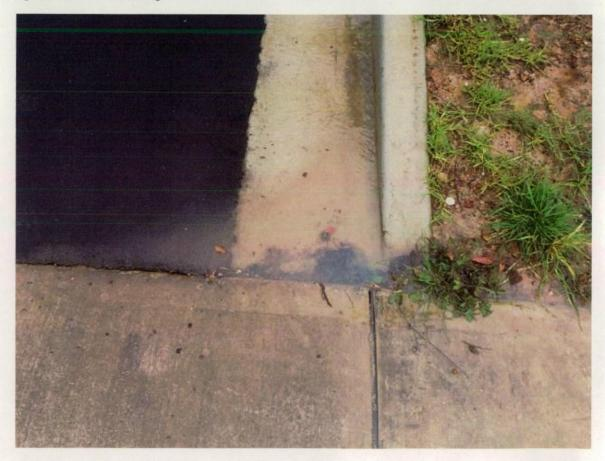
Figure 96 Gutter holding water.
