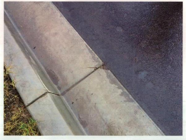
Figure 230 Damage to gutter lip.
