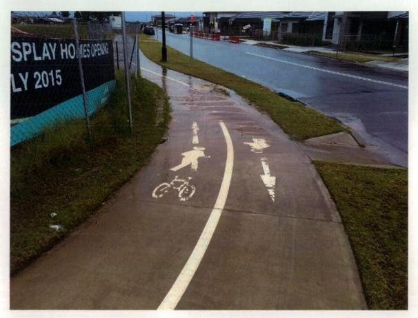
Figure 117 Damage to cycle way line marking.
