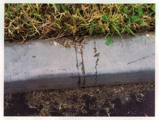
Figure 53 Cracks in kerb.
