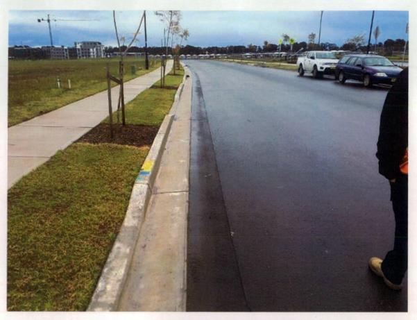
Figure 413 Surface marks on K&G and marks in asphalt.
