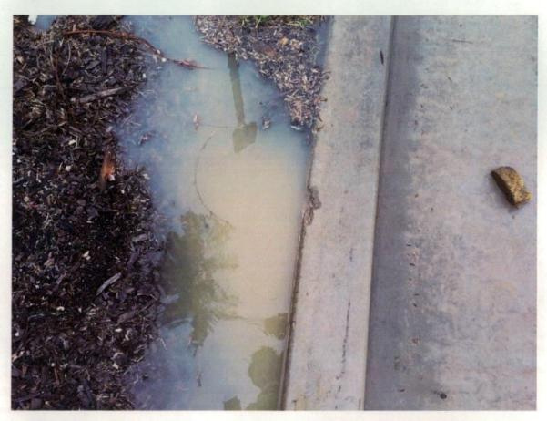
Figure 109 Holding water in footpath area.
