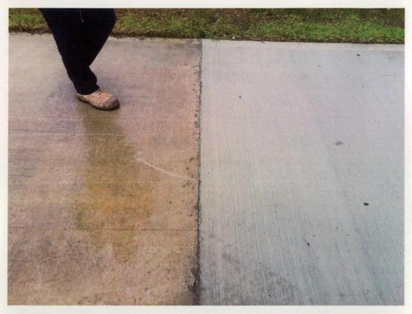
Figure 23 Concrete stains at path joint.
