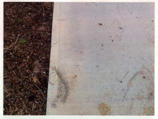
Figure 506 Concrete splatter on footpath.
