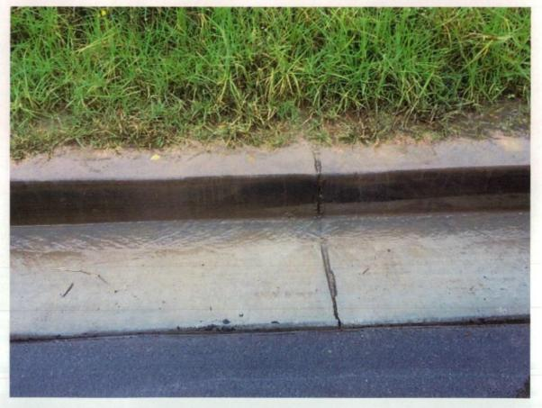
Figure 168 Staining to kerb.
