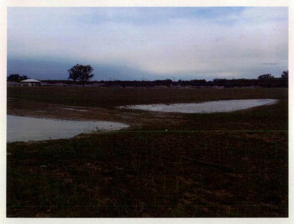
Figure 447 Holding water in low spots on site.
