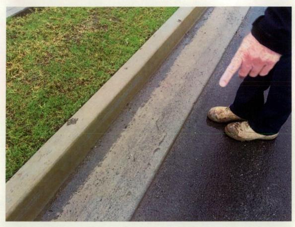
Figure 268 Surface imperfections on gutter.
