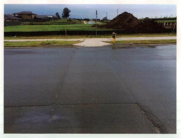
Figure 246 Asphalt has uneven finish.
