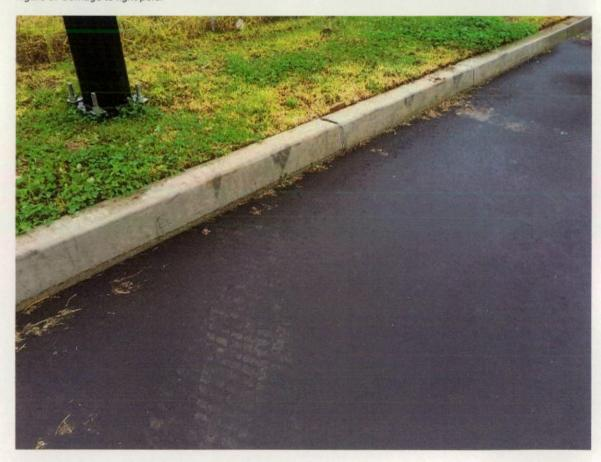
Figure 68 Tyre marks on asphalt and kerb.
