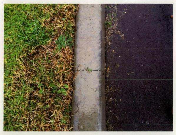
Figure 55 Crack to kerb.
