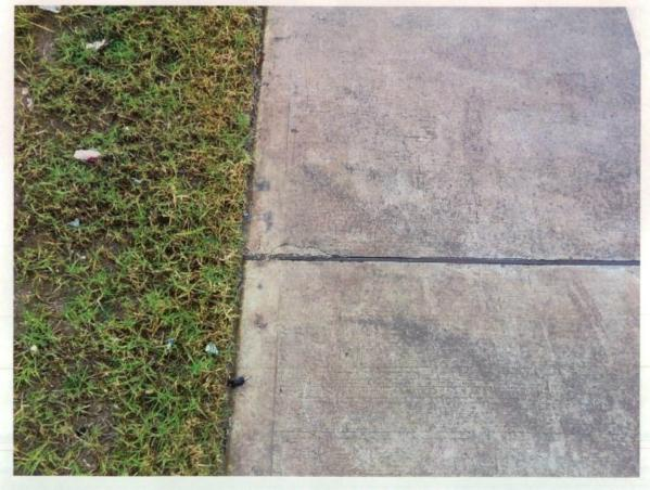
Figure 144 Cracks in footpath surface.
