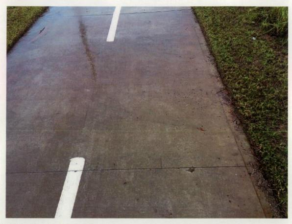
Figure 141 Damage to footpath surface.
