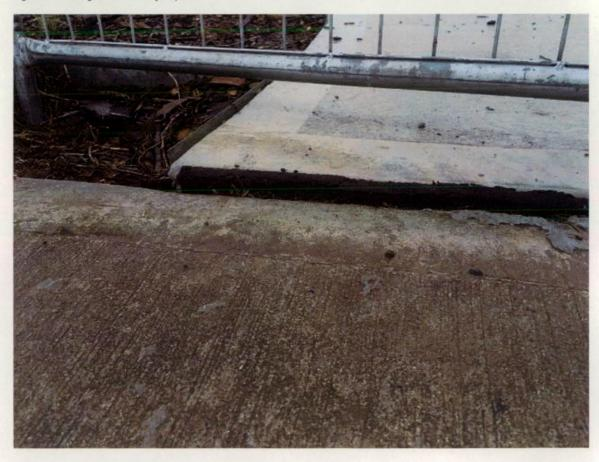
Figure 12 Poor interface between concrete footpaths.
