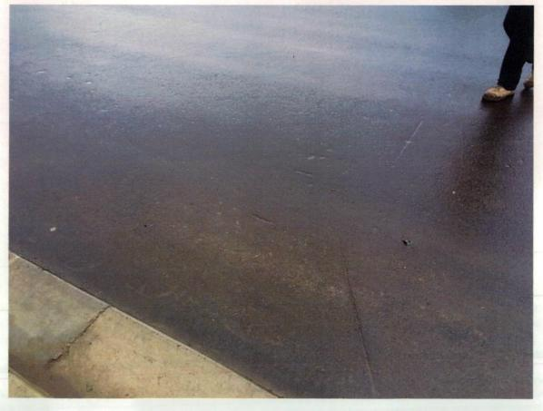
Figure 212 Staining and surface marks on asphalt.
