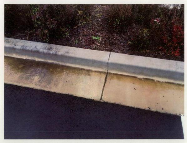
Figure 59 Bitumen stain on kerb.
