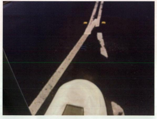
Figure 406 Damage to round about line marking.
