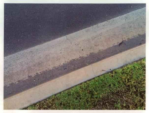
Figure 266 Crack in K&G.
