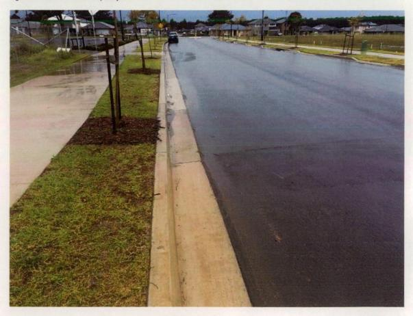
Figure 24 Concrete splatter and marks on K&G, asphalt surface marked.
