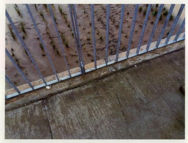
Figure 3 Wide gaps at expansion joint and crack on bridge.
