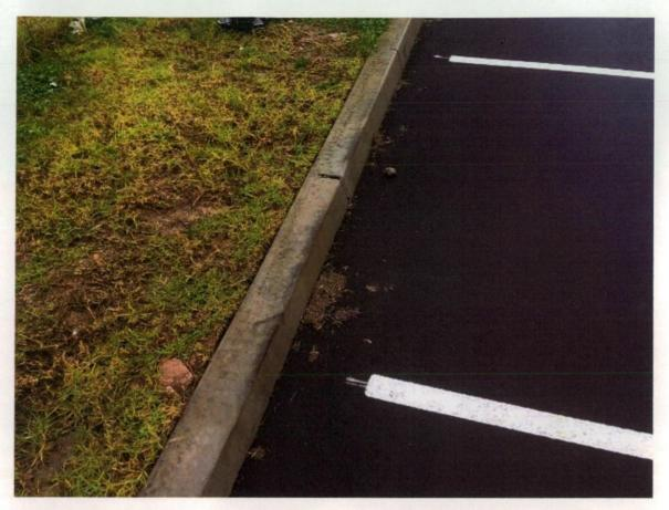
Figure 81 Staining and damage to kerb.
