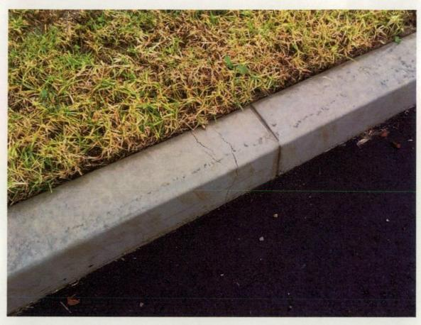
Figure 79 Crack in concrete kerb.
