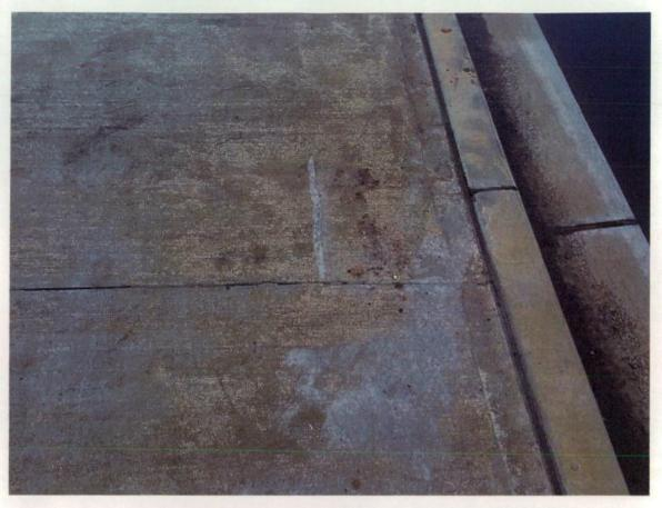
Figure 5 concrete splatter and staining present
