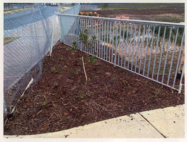
Figure 448 Fence damaged and mulch untidy in garden bed.
