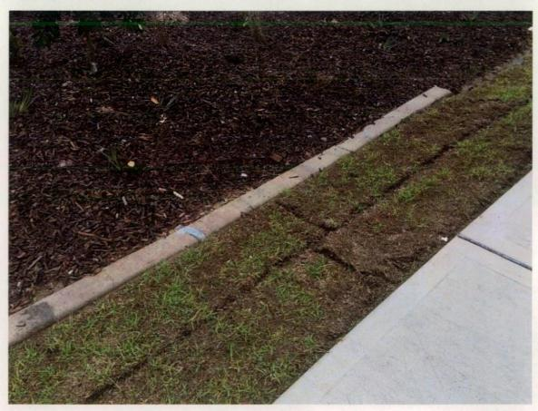
Figure 360 Damage to concrete edge.
