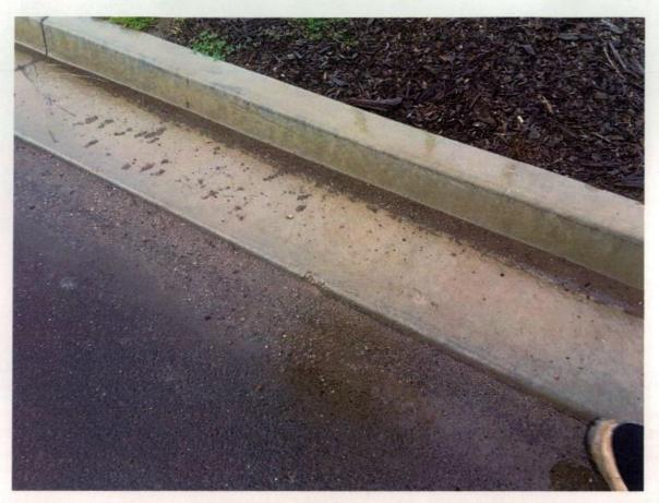
Figure 255 damage to kerb lip.
