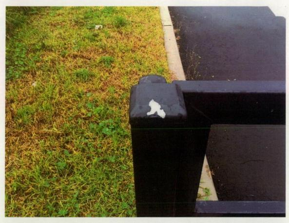
Figure 39 Paint Missing on boom gate.
