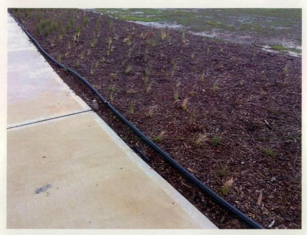
Figure 455 Broken temporary irrigation.
