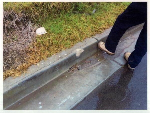
Figure 172 Patching on kerb.
