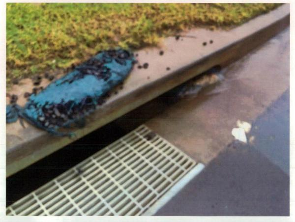
Figure 410 Existing silt control, breaking up and going down the drain.
