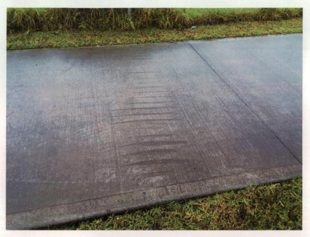
Figure 278 Machinery has damaged footpath surface.
