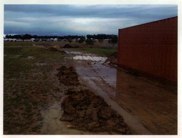
Figure 441 Holding water in wheel ruts.
