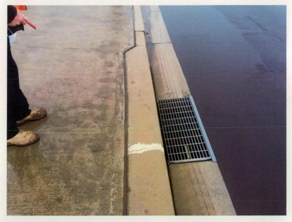
Figure 7 Crack repaired in lintel
