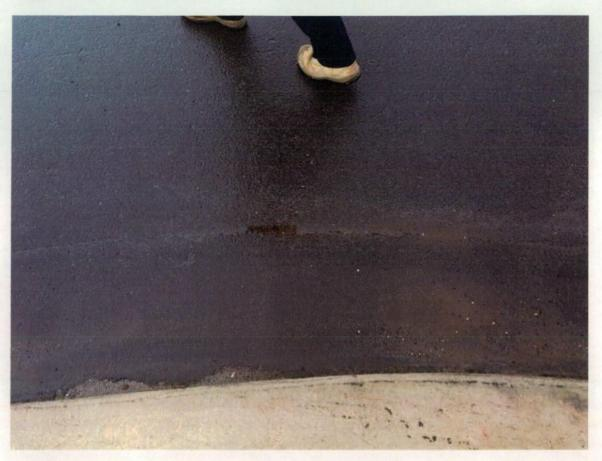
Figure 397 surface imperfections in asphalt edge.
