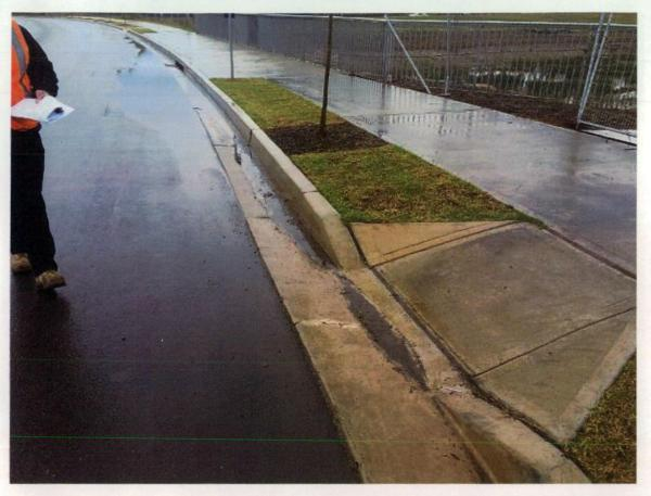
Figure 13 Kerb crack repair on pram ramp.
