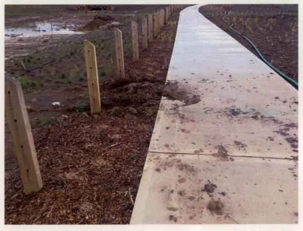
Figure 504 Wheel ruts and excess soil on concrete footpath.
