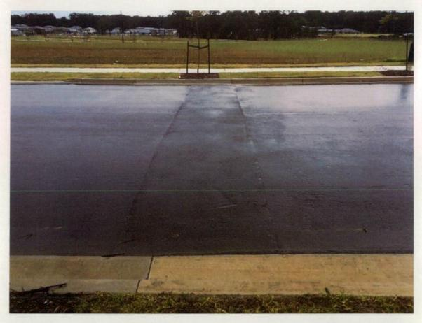
Figure 27 Uneven road surface due to trenching.
