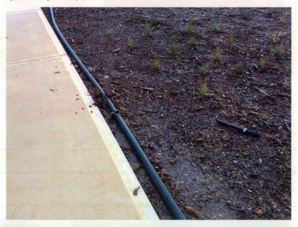
Figure 490 Broken existing irrigation main.
