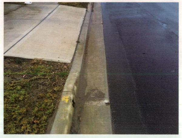
Figure 382 Cracks in K&G and egress of silt runoff.
