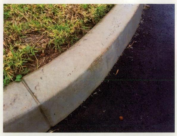
Figure 71 Chips to concrete kerb.
