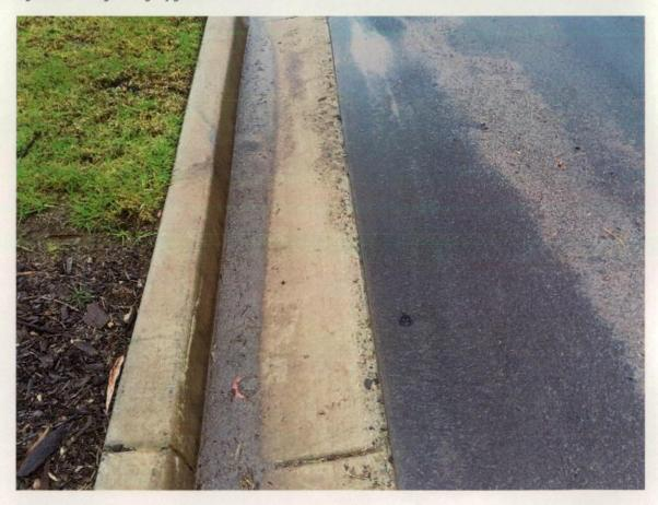
Figure 325 Damage to the lip of gutter.
