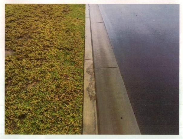
Figure 132 Patching work to kerb.
