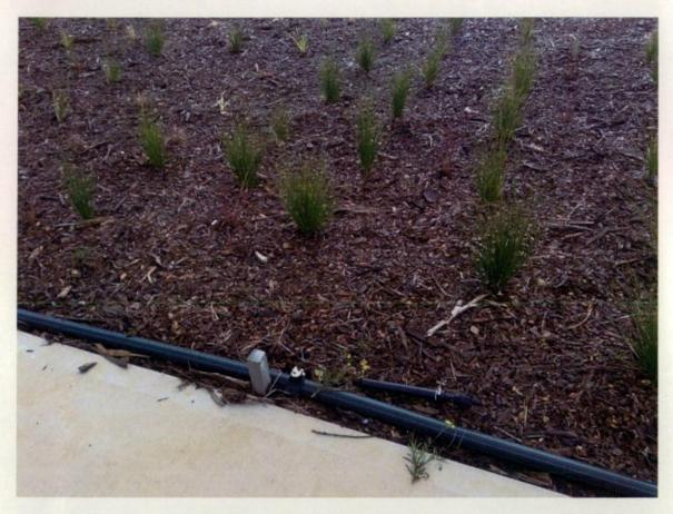
Figure 459 Broken temporary irrigation system.
