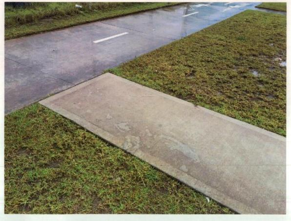
Figure 136 Concrete stains to footpath.
