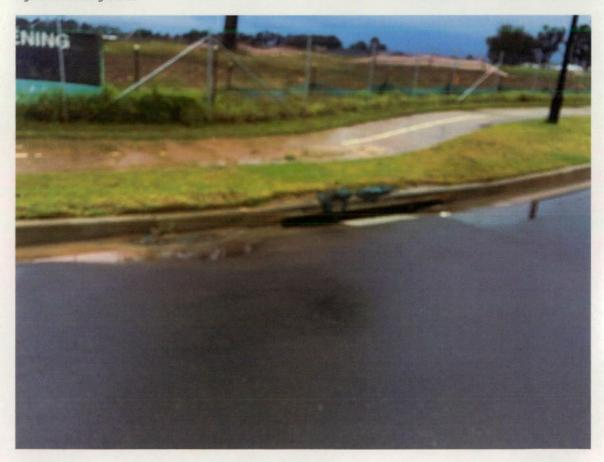
Figure 408 Existing silt control, breaking up and going down the drain.
