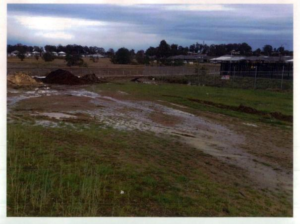
Figure 446 Wheel ruts holding water, stockpiled materials.
