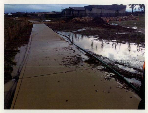
Figure 487 Holding water in garden bed, wheel ruts and stockpiles of construction waste.
