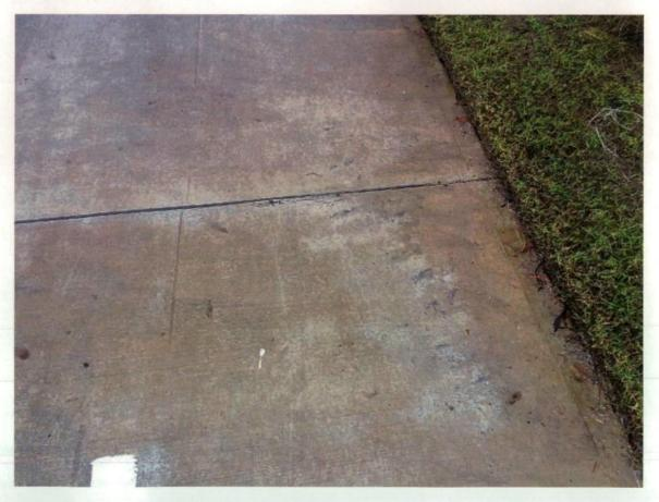
Figure 140 Scratches and damage by machinery to footpath.
