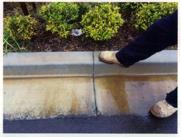
Figure 46 Cracking in kerb, wide crack in joint.
