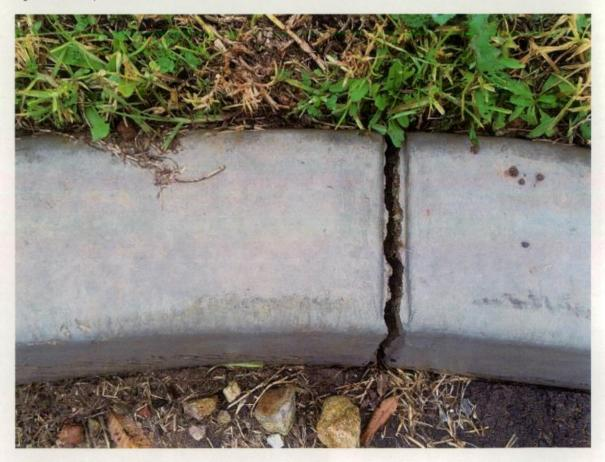
Figure 52 Wide crack present on joint.
