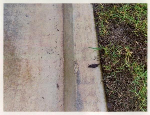
Figure 28 Chips in kerb.
