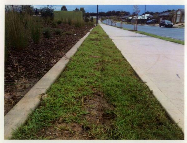
Figure 351 Wheel ruts in turf, damage to concrete garden edge.
