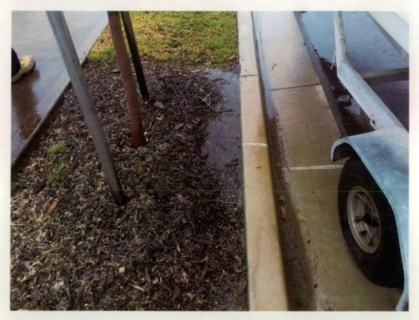
Figure 320 Holding water in low area.
