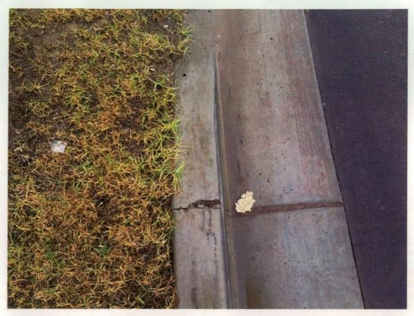
Figure 207 Damage to kerb joint.
