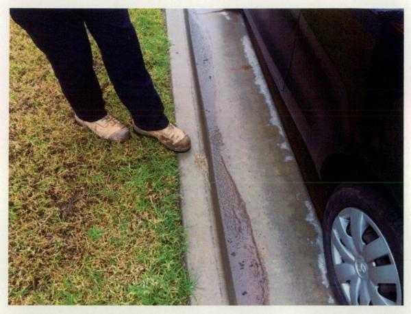
Figure 328 Damage to kerb and patching on gutter.
