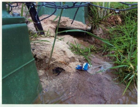
Figure 156 Sand around electrical service boxes washed away.
