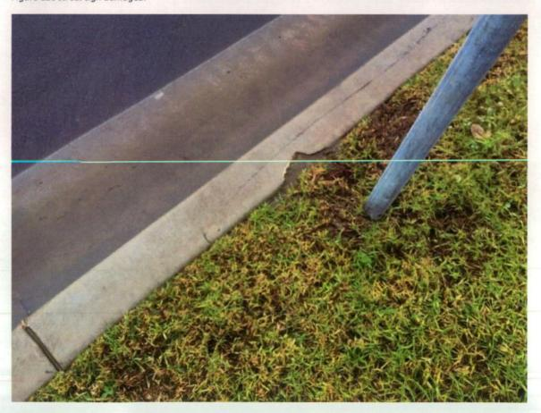
Figure 129 Chips to back of kerb.
