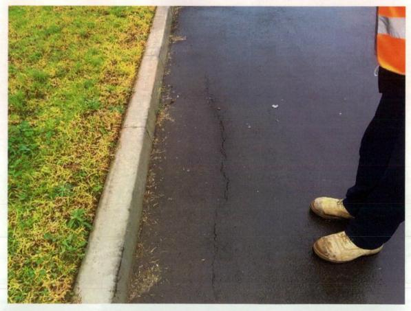
Figure 54 Cracks in carpark asphalt.
