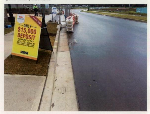
Figure 400 Edge damage and existing construction barriers.
