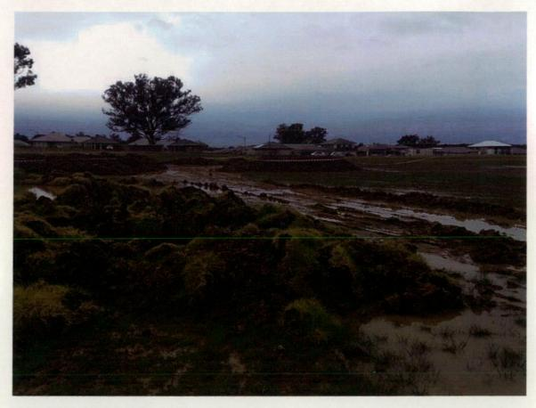
Figure 439 Soil stockpiled, wheel ruts holding water.
