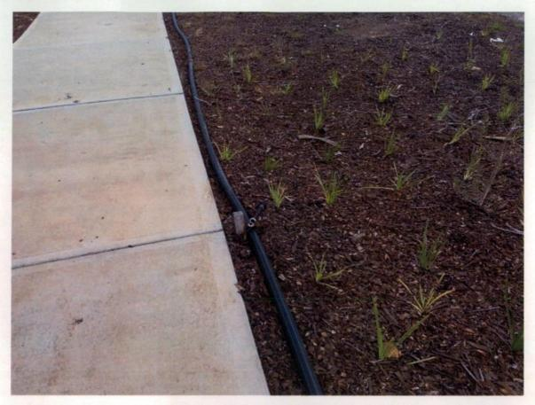
Figure 453 Broken temporary irrigation.
