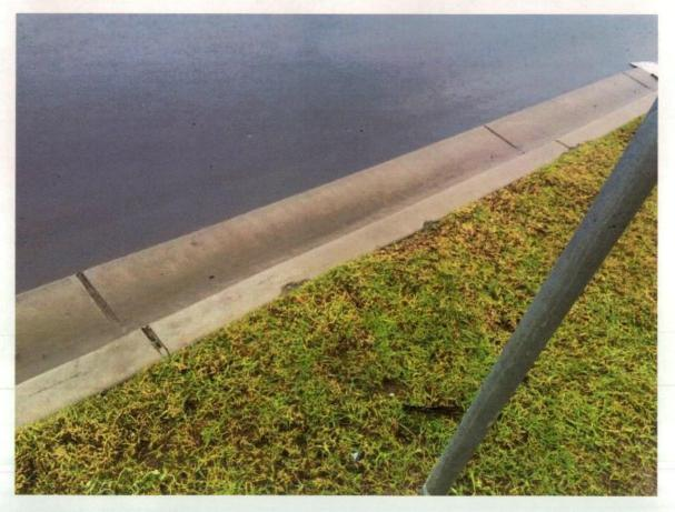
Figure 126 Chips to back of kerb.
