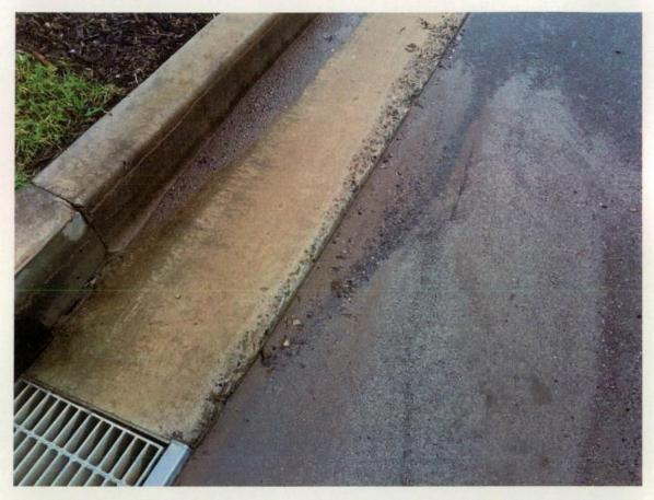
Figure 324 Damage to edge of gutter.
