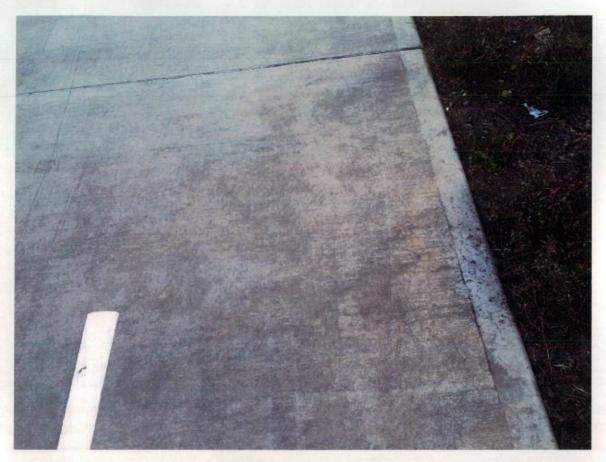
Figure 97 Stain on concrete footpath.
