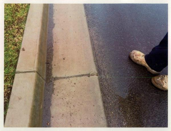
Figure 272 Damage at concrete joint.
