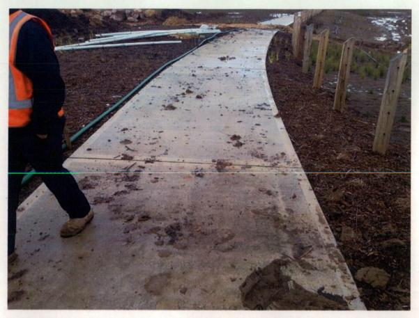
Figure 505 Excess soil on concrete footpath.
