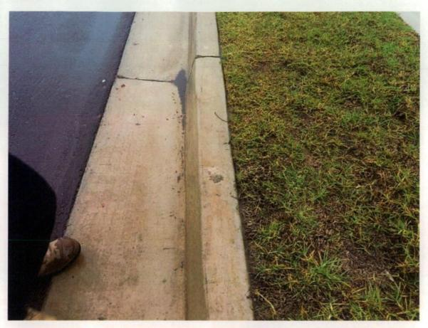
Figure 29 Concrete splatter on kerb.
