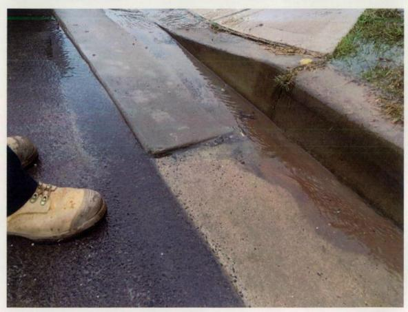
Figure 162 Lintel and pram ramp at different level.
