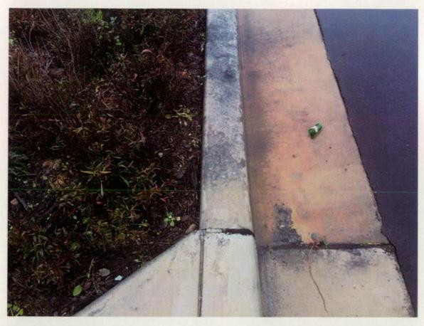
Figure 91 Damage to kerb and pram ramp.
