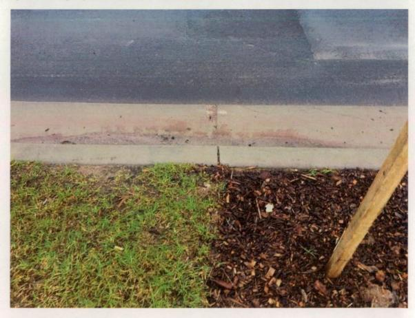
Figure 376 Silt runoff into K&G
