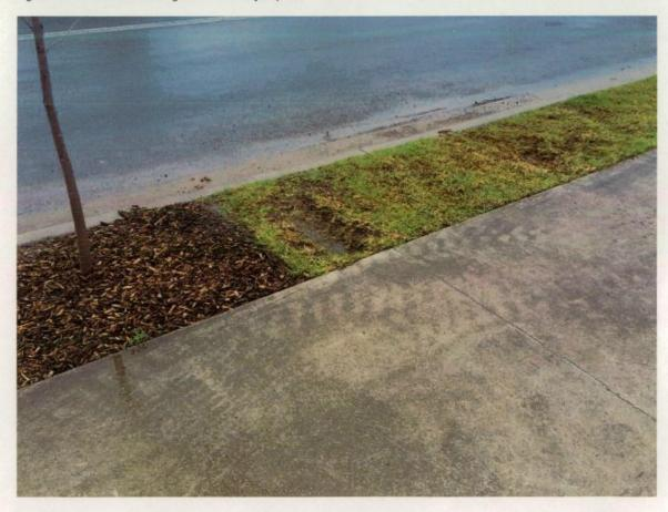
Figure 380 Wheel ruts in turf area.
