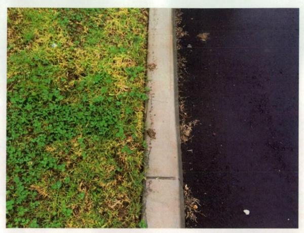
Figure 73 Staining and surface cracking to kerb.
