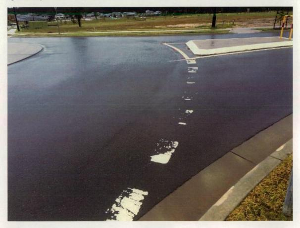
Figure 116 Line marking worn away.
