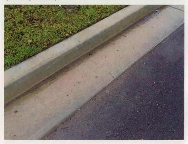
Figure 254 Crack in K&G.
