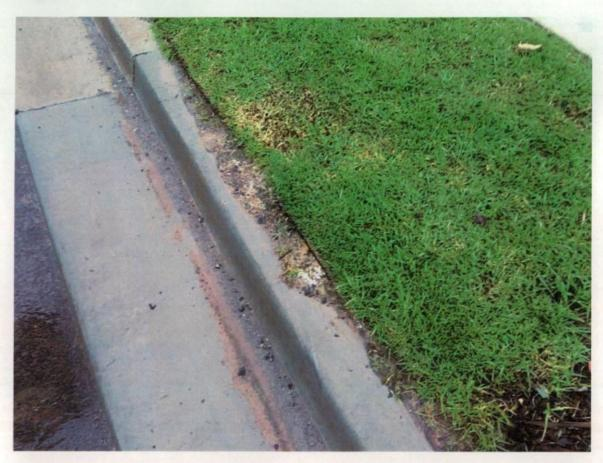
Figure 349 Clay/soil runoff into gutter.
