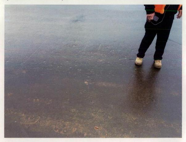
Figure 206 Pitting on asphalt surface.
