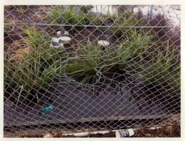
Figure 507 Chain link fence damaged.
