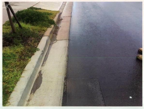
Figure 398 Existing silt and gutter damage opposite site.
