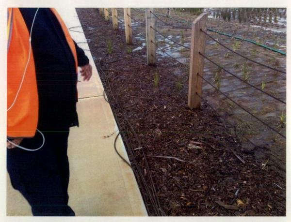
Figure 483 Cables cut from handrail near riparian
