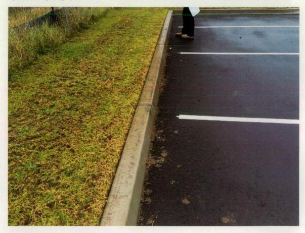
Figure 84 Damage and concrete splatter on kerb.
