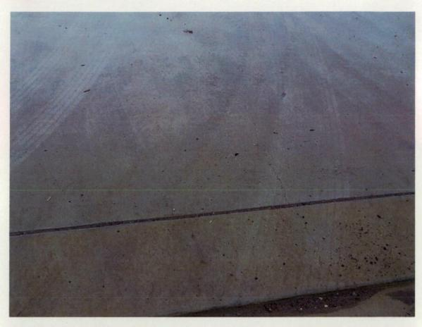
Figure 367 Tyre marks and cracks on substation driveway.
