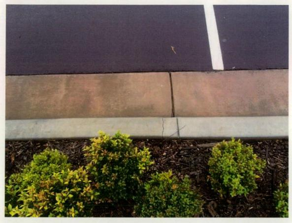
Figure 99 Crack in kerb.
