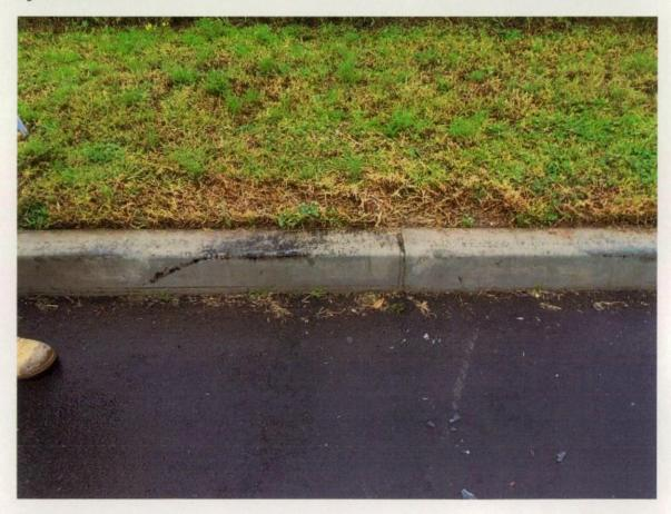
Figure 56 Bitumen stains to kerb.
