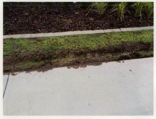
Figure 368 Wheel ruts in turf area.
