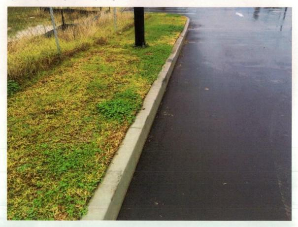
Figure 62 Marks on kerb from machinery.
