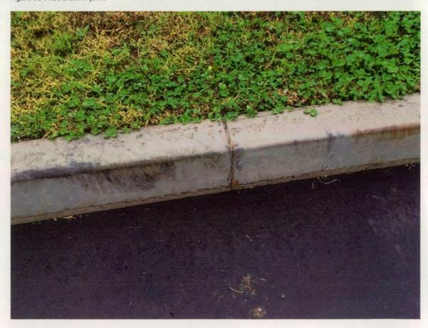
Figure 64 Staining to kerb.
