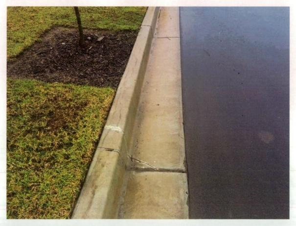
Figure 102 Crack that has been repaired in K&G.
