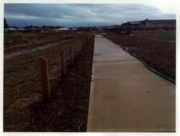
Figure 477Steel cables from handrail cut and on footpath.
