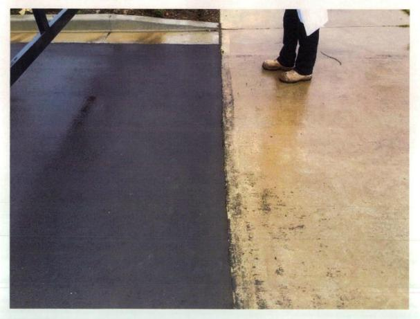
Figure 38 Bitumen staining on concrete surface.
