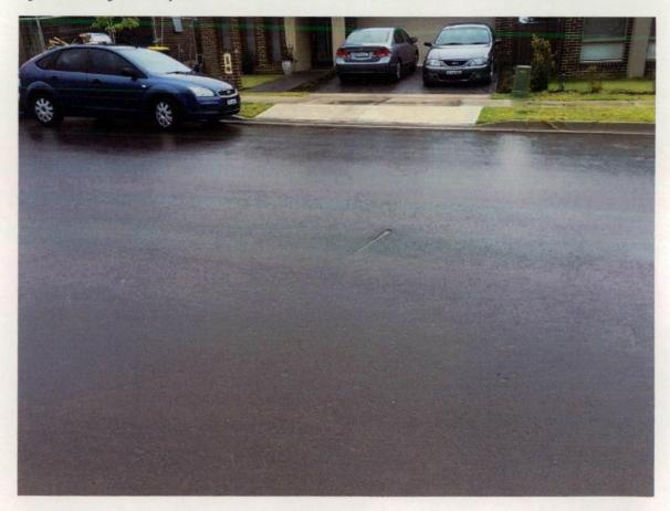
Figure 222 Gouge in asphalt surface.
