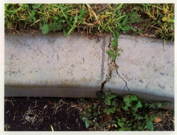
Figure 51 Cracks present in kerb.
