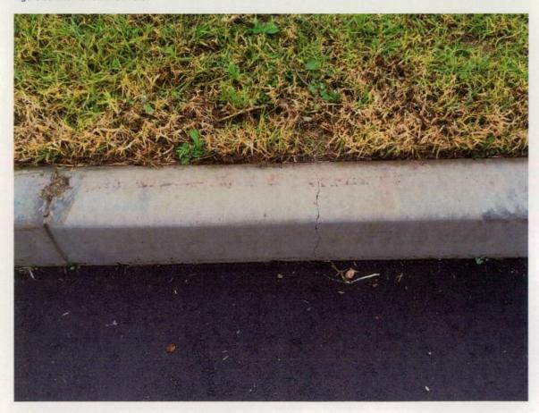
Figure 60 Crack in kerb.
