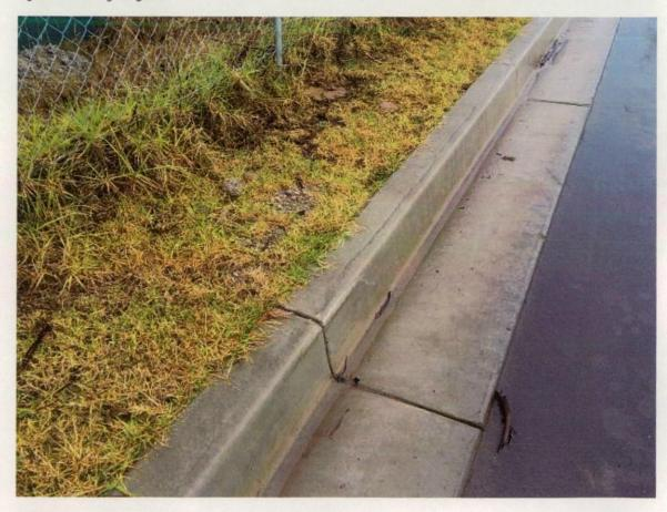
Figure 182 Surface stains on kerb.
