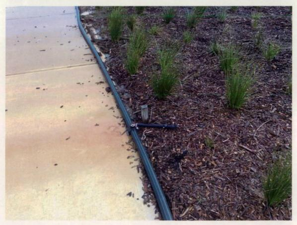
Figure 460 Broken temporary irrigation system.
