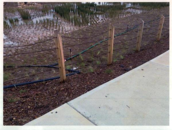
Figure 450 Loose wire on fence, existing irrigation system parts broken.
