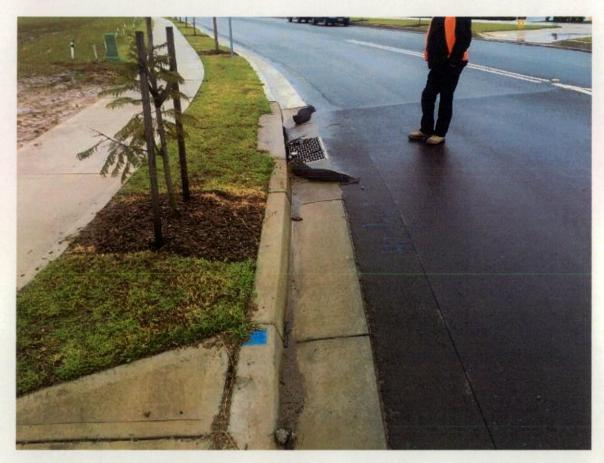
Figure 411 Existing silt and silt controls in gutter opposite site.
