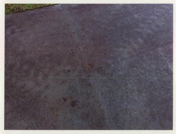
Figure 535 Cracks and wheel marks on pavement surface.
