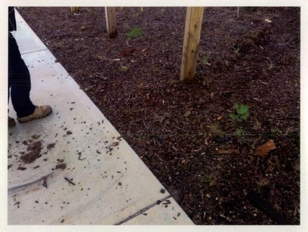
Figure 531 wheel ruts and marks on footpath.
