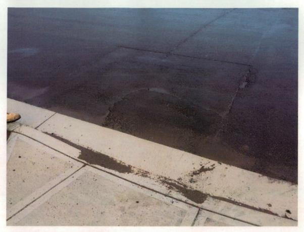
Figure 245 Asphalt has uneven finish.
