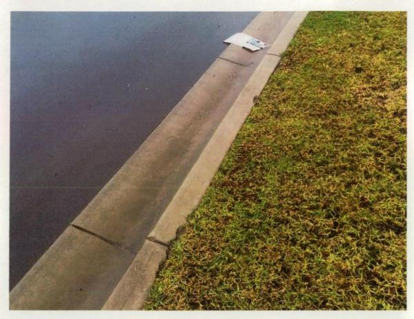
Figure 127 Chips to back of kerb.
