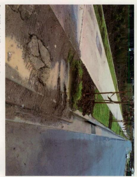
Figure 341 Wheel ruts holding waer at existing site access.
