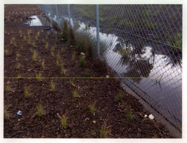
Figure 509 Holding water at low point.
