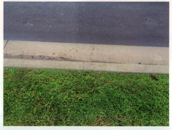
Figure 362 Crack in K&G.
