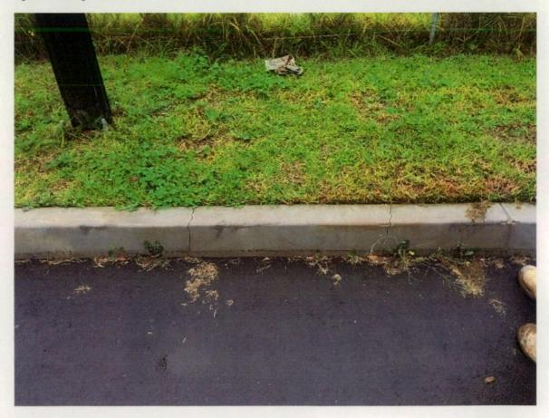
Figure 48 Cracks in kerb.
