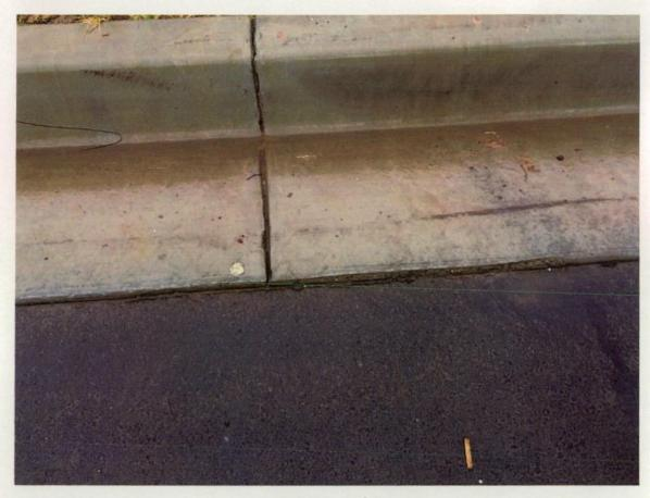
Figure 197 damage to gutter lip.
