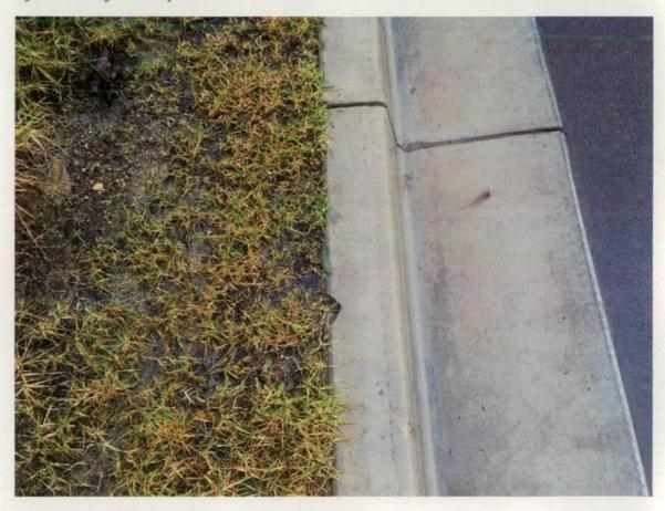
Figure 226 Damage on back of kerb.
