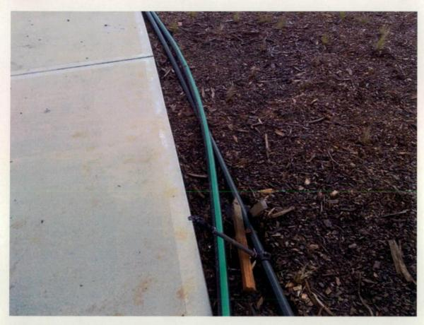
Figure 491 Broken existing temporary irrigation.
