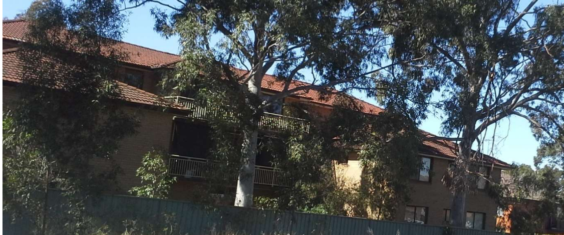
Figure 6.1: Windows and balconies to adjoining property at 8 Railway Street
