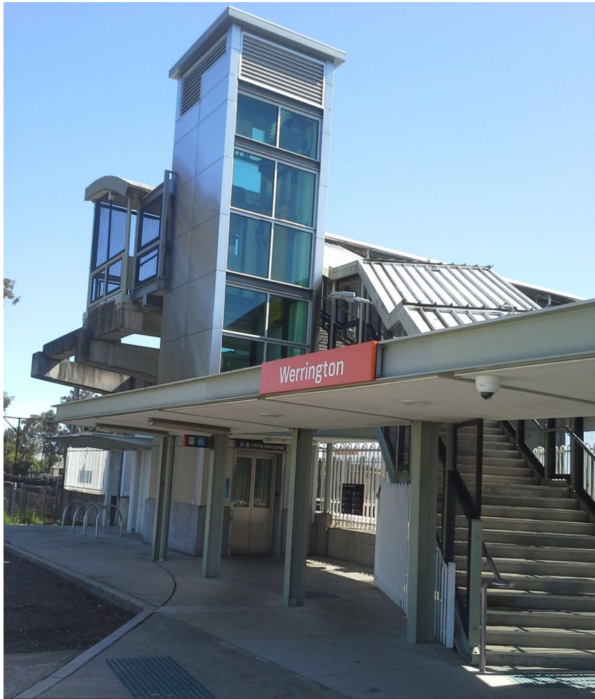
Figure 1.9: Werrington Railway Station showing disabled access
