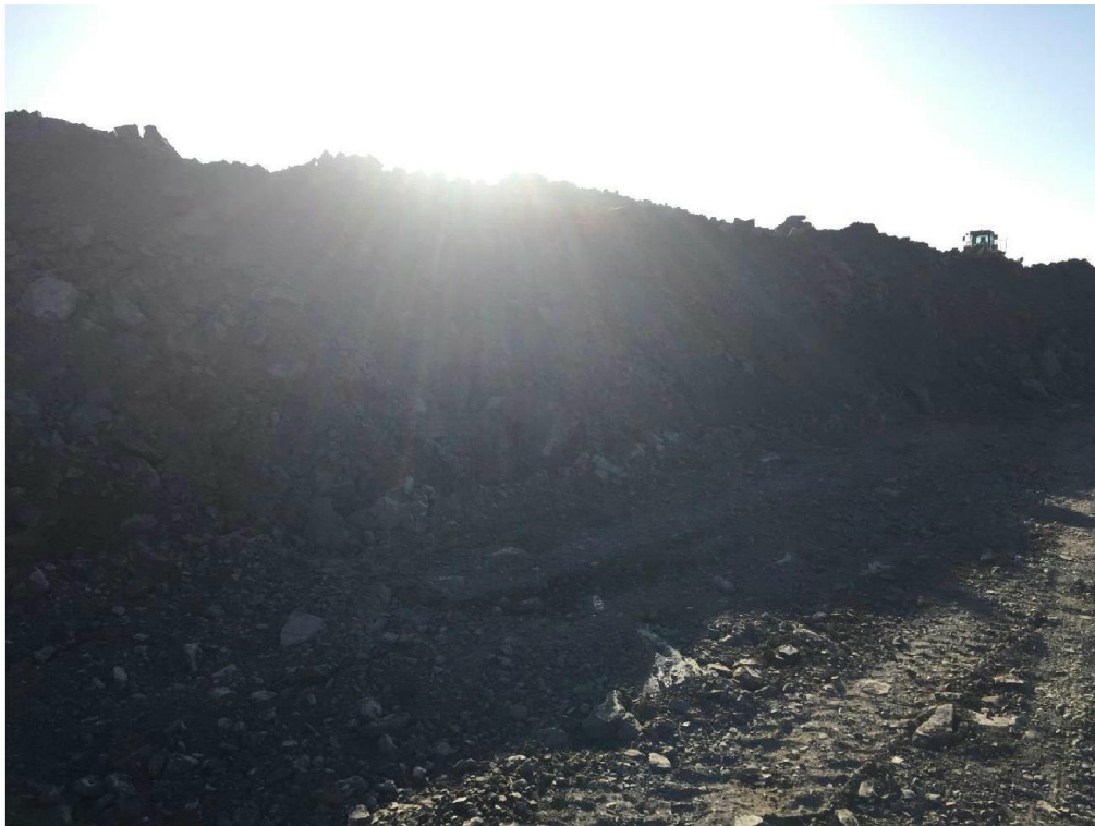
Stockpiled Shale being Loaded
