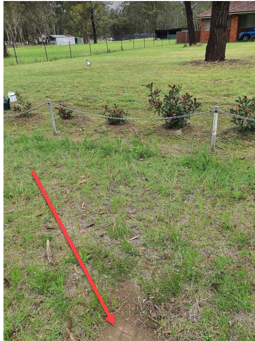
Photo 8: Hydrant located directly in front of existing dwelling.
