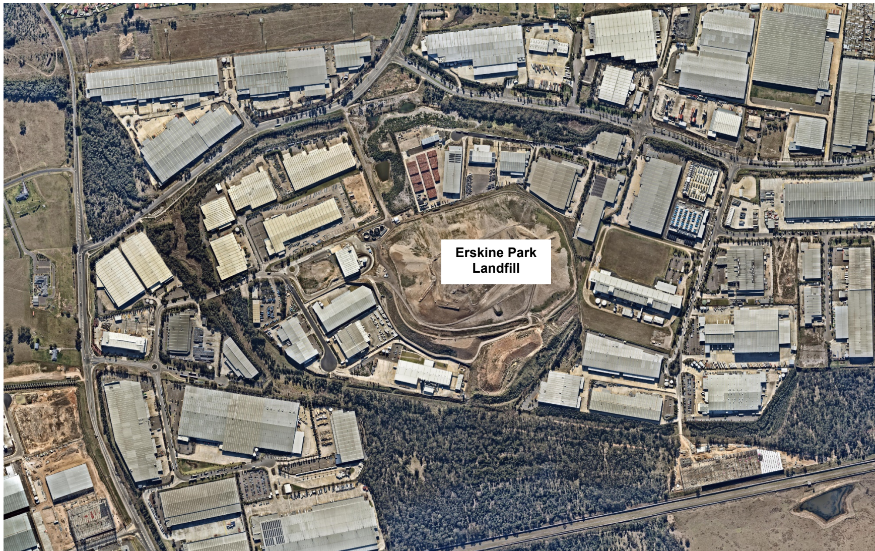
Figure 1: Site Location and Surrounding Land Usage (Source: Near Map image 20 July 2019)
