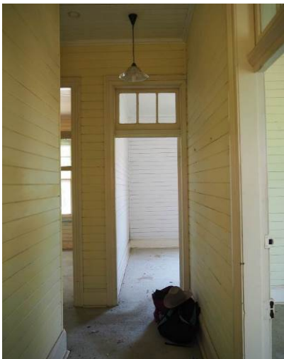
Figure 3. 62: S3 (entry hall) looking west from Front door to S2 (bedroom).
