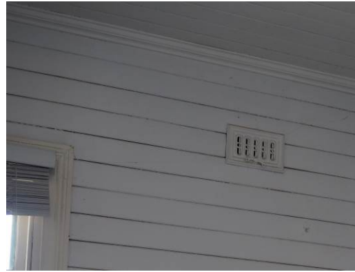
Figure 3. 87: Typical pressed metal air vent.
