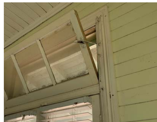
Figure 3. 85: Fanlight above door to S1.
