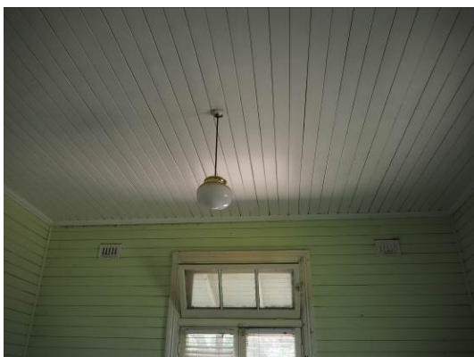
Figure 3. 82: Detail of timber boarded ceilings.
