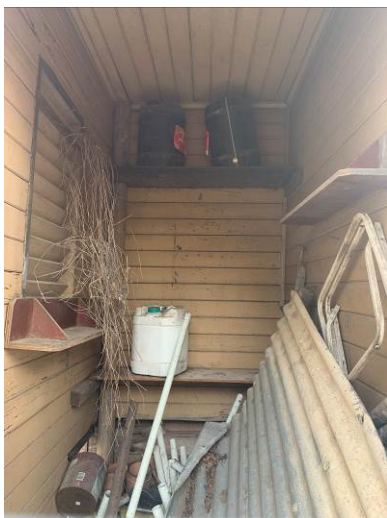
Figure 3. 95: Interior view of north space.
