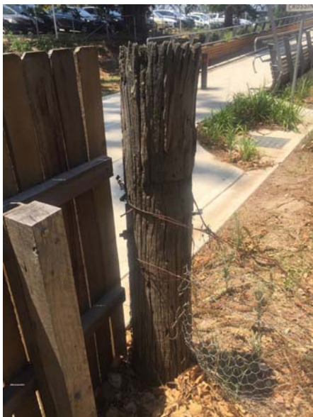
Figure 3. 32: A remnant timber post at Punt Road that forms the start of the earlier lot fence along the eastern site boundary. Note the strained wire and netting and the check for the missing timber straining brace.
