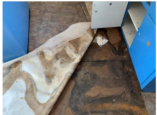
Figure 3. 78: Vinyl floor covering in S9 (kitchen).
