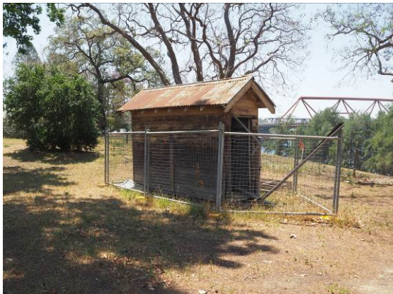
Figure 3. 91: West and south elevations.
