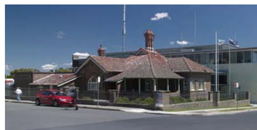
Figure 4. 5: Armidale Police Station Source: http://mcintoshphelps.com.au/portfolio
