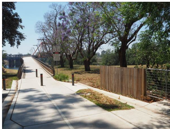
Figure 3. 3: view looking east along shared pathway to the pedestrian bridge crossing over the Nepean River.
