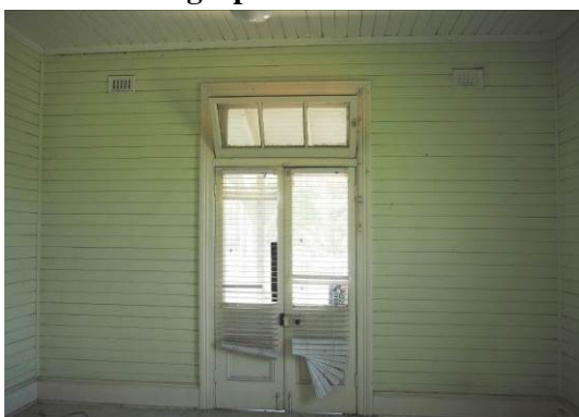
Figure 3. 58: S1 (bedroom) with French door leading to north (front) verandah.
