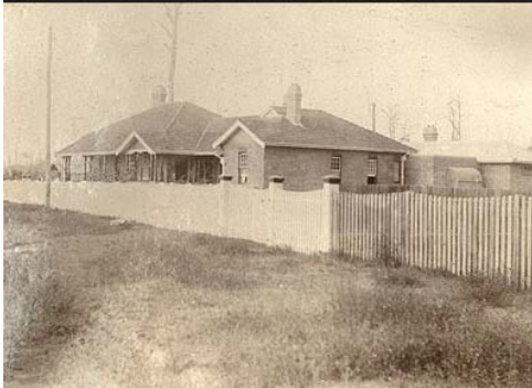
Figure 4. 1: Macksville Courthouse and Police Station. Source: NSW State Archives/ 4346_a020_a020000311
