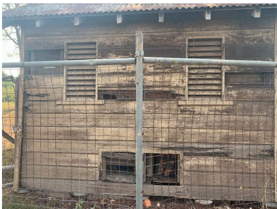
Figure 3. 93: East elevation with louvered openings and access openings for cans.
