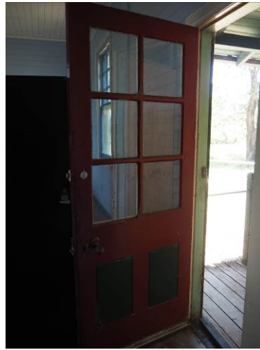
Figure 3. 89: Door D5 (door from kitchen to south verandah).
