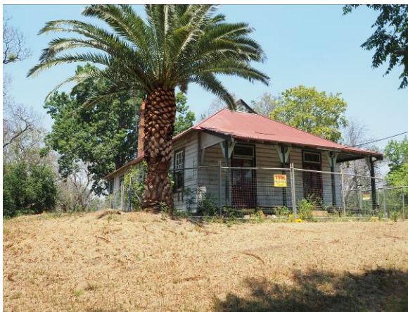
Figure 3. 8: The street frontage of the former Police Residence property in its landscaped setting.
