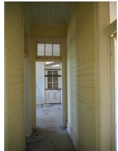
Figure 3. 64: S3 (entry hall) looking south towards living room.
