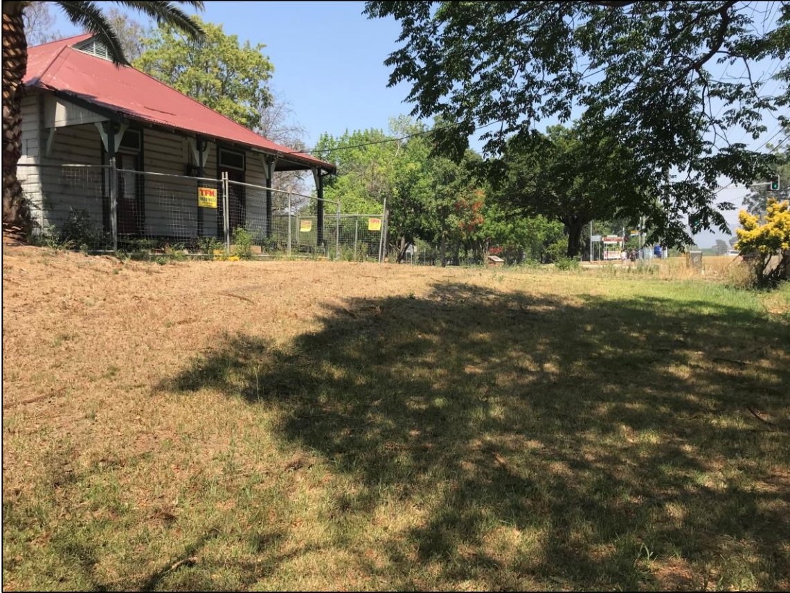
Photograph 5: Showing the front yard of the former Police residence.
