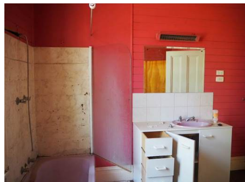
Figure 3. 66: S4 (former bedroom) with bathroom fitout
