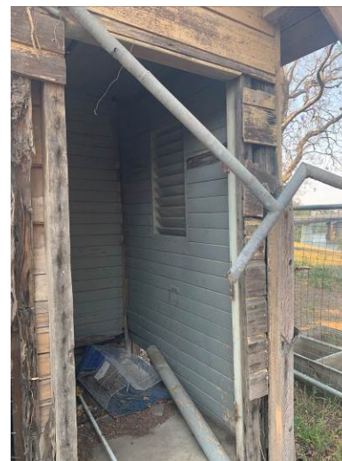
Figure 3. 97: Interior view of south space.
