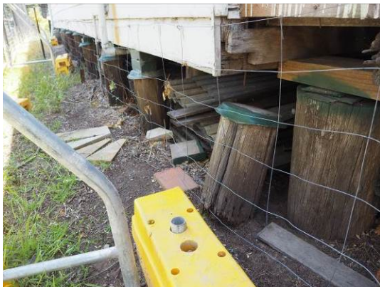
Figure 3. 53: Timber log piles with ant caps.
