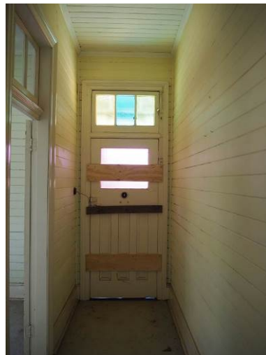
Figure 3. 63: Internal view of Front door on east elevation.
