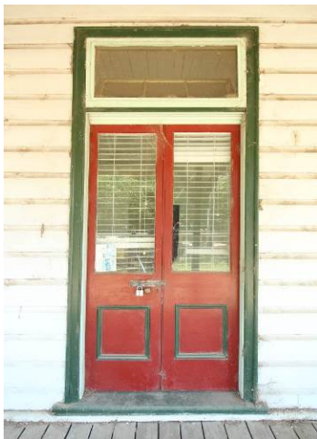
Figure 3. 55: Door to northern elevation.
