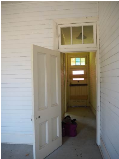
Figure 3. 88: Typical internal door with fanlight.
