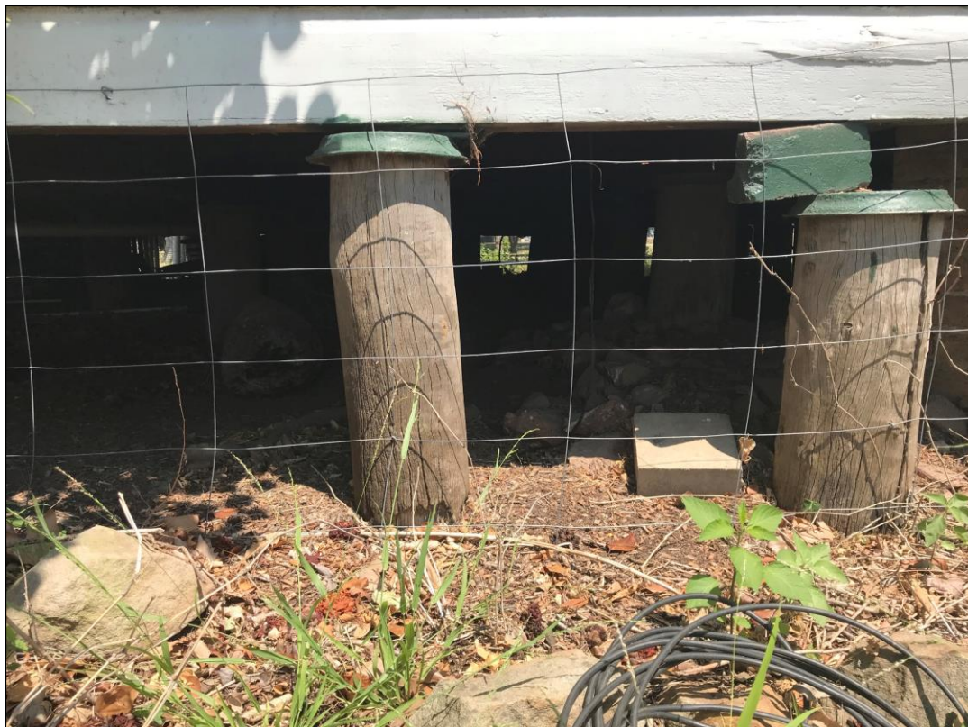
Photograph 2: Showing the footings of the former Police residence.
