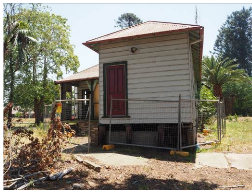
Figure 3. 44: South (rear) elevation of east wing extension.
