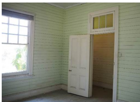
Figure 3. 59: S1 (bedroom) door with fanlight and window.
