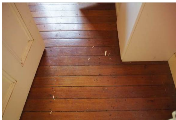
Figure 3. 83: Timber floor to S4 (bathroom).
