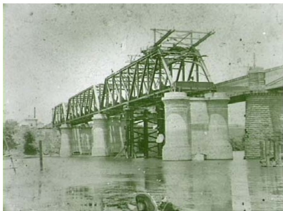
Figure 2. 22: 1906 photograph of the Victoria Bridge and the rail bridging under construction. Source: Penrith City Council, 608
