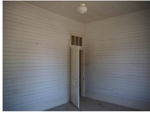
Figure 3. 61: S2 (bedroom) door with fanlight and vee-jointed panelled walls.
