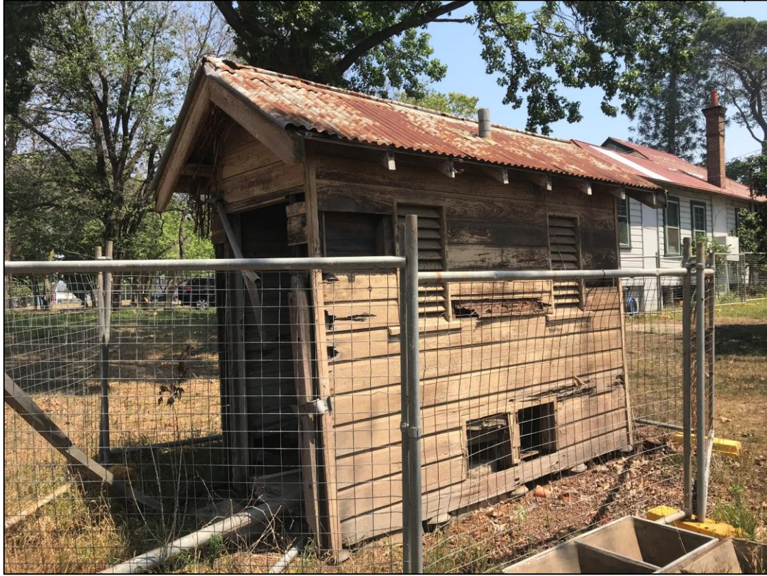
Photograph 3: Showing the extant timber outbuilding.
