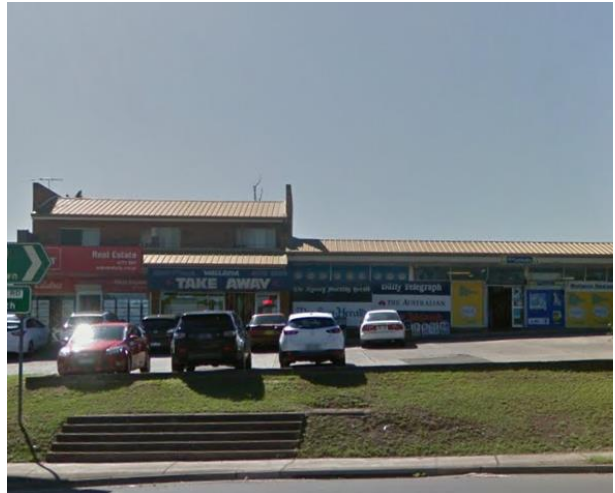
Picture 8 – Wallacia Shops, Mulgoa Road Source: Google Earth
