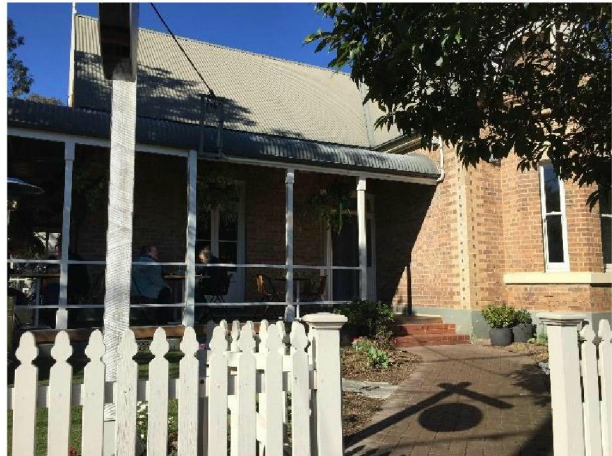
Figure 12 – Verandah on west elevation, 146 Station Street
