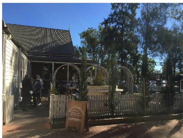
Figure 10 – Rear dining courtyard, Percy Plunkett Café, 146 Station Street
