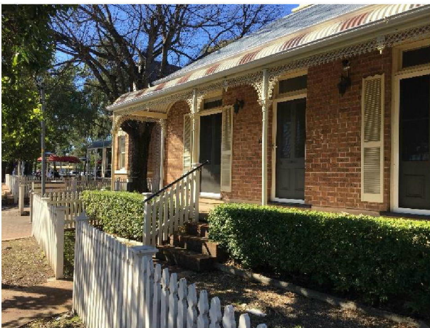
Figure 17 – Front (west) elevation, 148 Station Street looking north. Shows small front garden with picket fence
