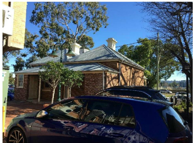
Figure 20– Rear (north east) elevation, 148 Station Street
