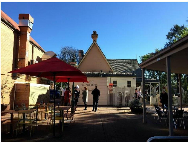
Figure 7 – View west showing courtyard at rear and side of 146 and 148 Station Street respectively
