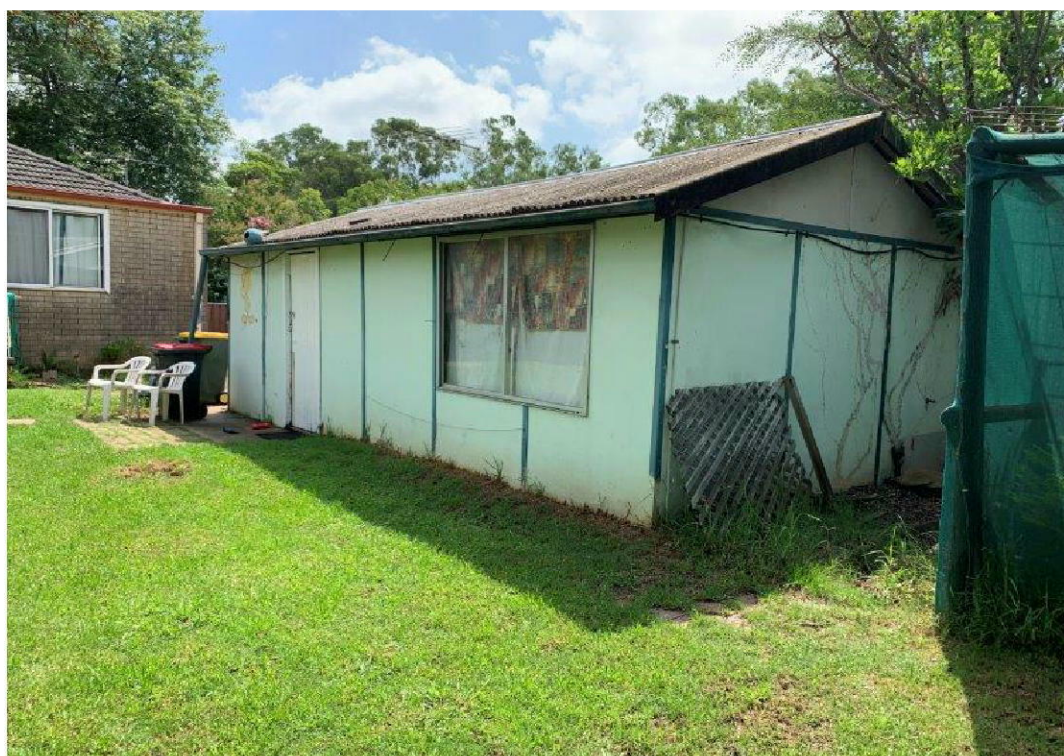
Photo 2 - 38 Orth Street, Fibre cement garage possibly containing asbestos cement
