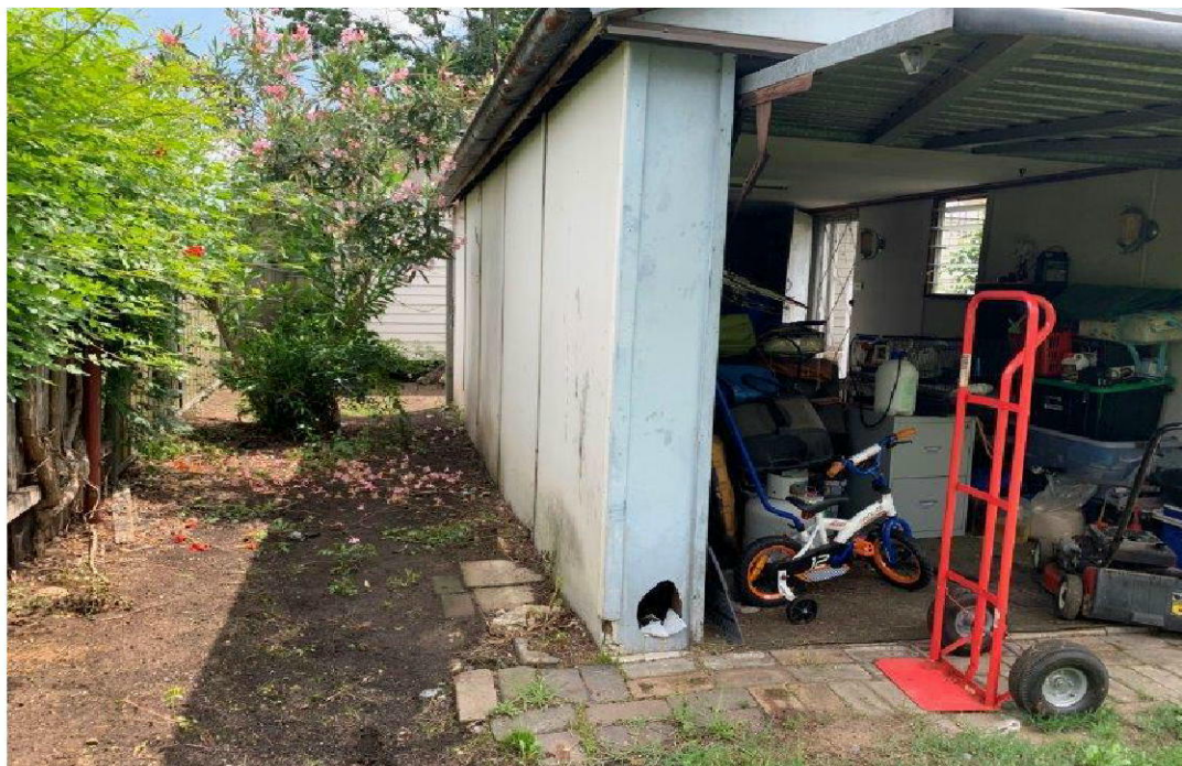
Photo 7 - 40 Orth Street, fibre cement garage with hole in wall
