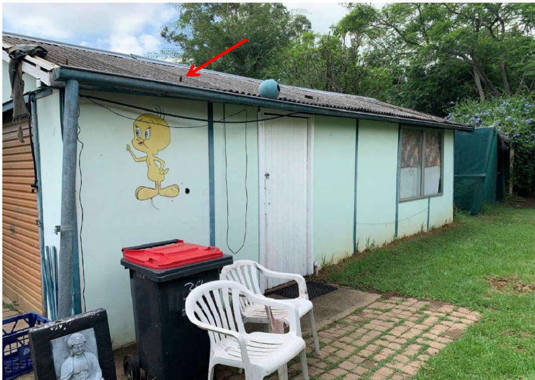
Photo 3 - 38 Orth Street, Cracks in fibre cement wall of garage and potential asbestos cement roof sheeting
