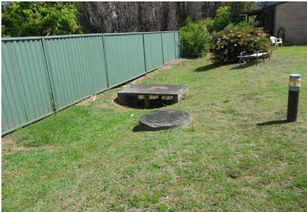
Photo 6 - Underground sewer or water pipes along southern boundary of the site
