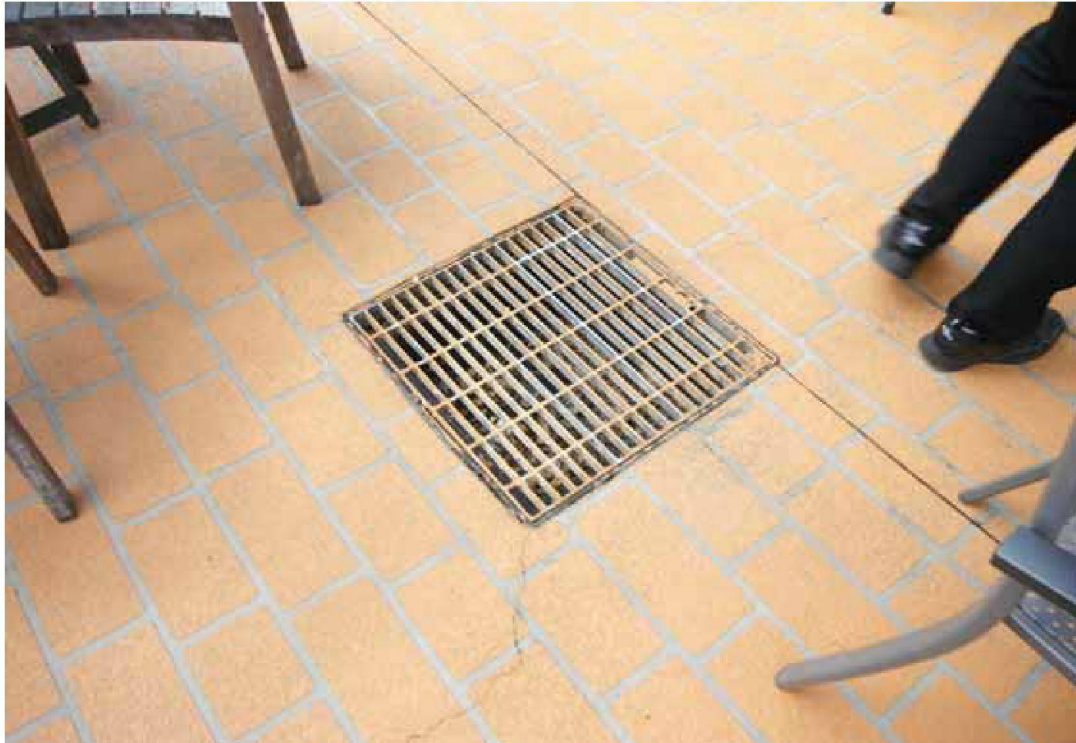
Photo 5 - One of many stormwater drains observed across the site. This drain located in central courtyard.
