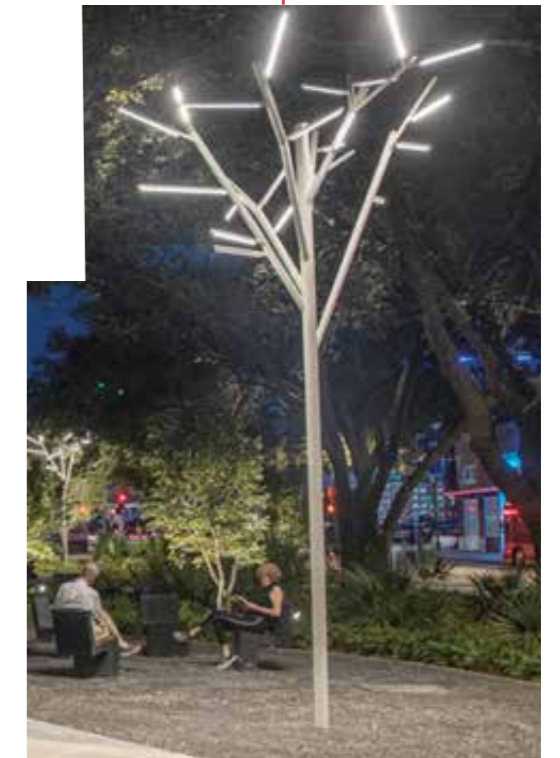
Light poles within grove of trees
