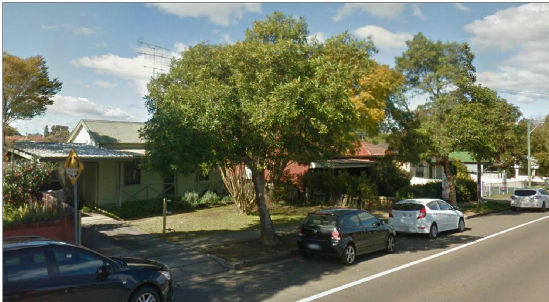
Figure 4: 28 Evan Street looking south (Source Google.com)
